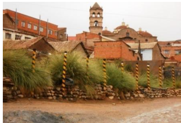
New construction without clear regulations for the conservation of the traditional urban image is affecting the Ribera de los Ingenios.
