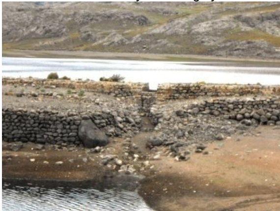
Water pipe in the Kari Kari hydraulic complex.
