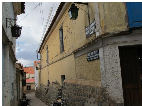
Traditional residence architecture with stone foundations and solid walls of adobe, December 2013
