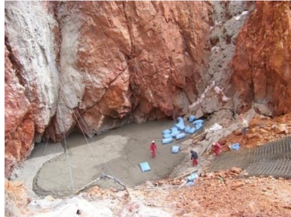
Filling works. Photo Empresa Q & Q.
