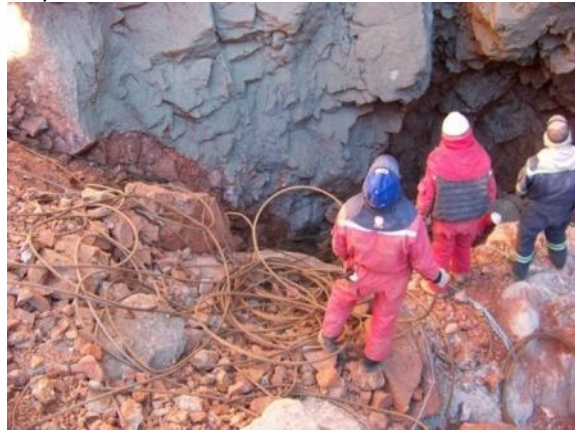
Revision of the collapse. Photo Empresa Q & Q.
