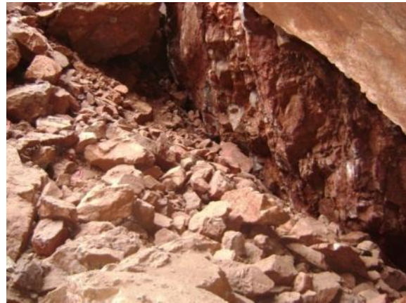
Separation of the filling of light concrete and the inside of the sinking.
