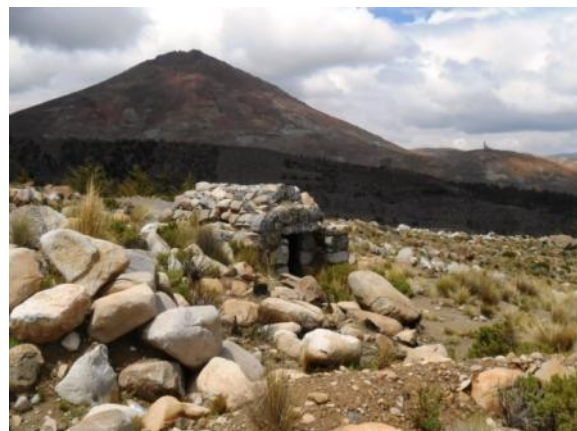
A water box that controls the flow of the fluid into the city of Potosí.
