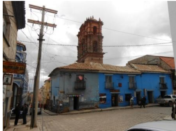
Cables that affect the perception of the monuments of the site.
