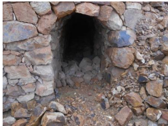
Appearance of an entrance to the mines located about 4,400 m. that continue operating.
