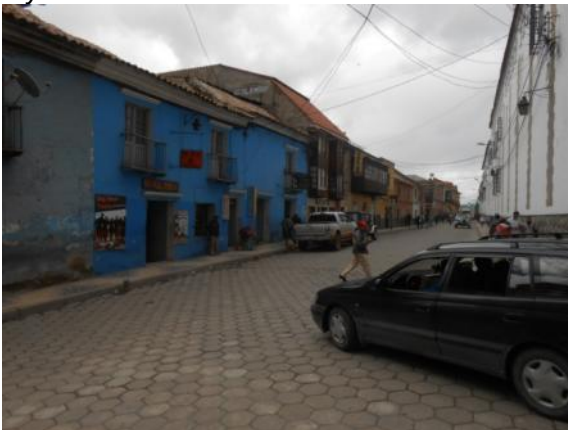
Pavement of concrete molded forms in one of the Potosí streets.
