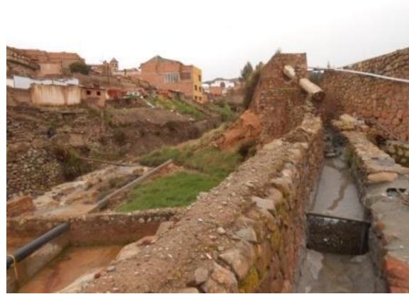
Historic water channel that still feeds some mining installations from the Kari Kari lagoons.
