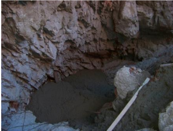
Start of the work for filling gaps. Photo Empresa Q & Q.
