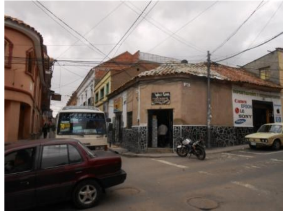
Visual contamination by cables and installations at the historic centre.
