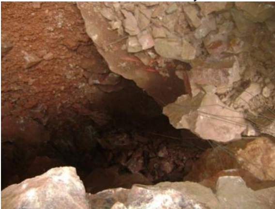
Inner aspect of the cavity under the filling of concrete lightened.
