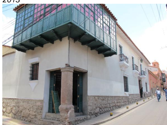
Wooden and glass balcony that acts as protection against the climate, December 2013
