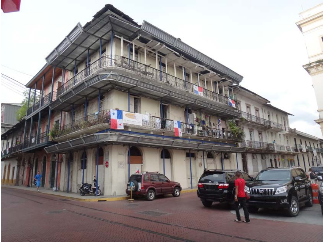
Restoration of historic buildings in the Historic District.
