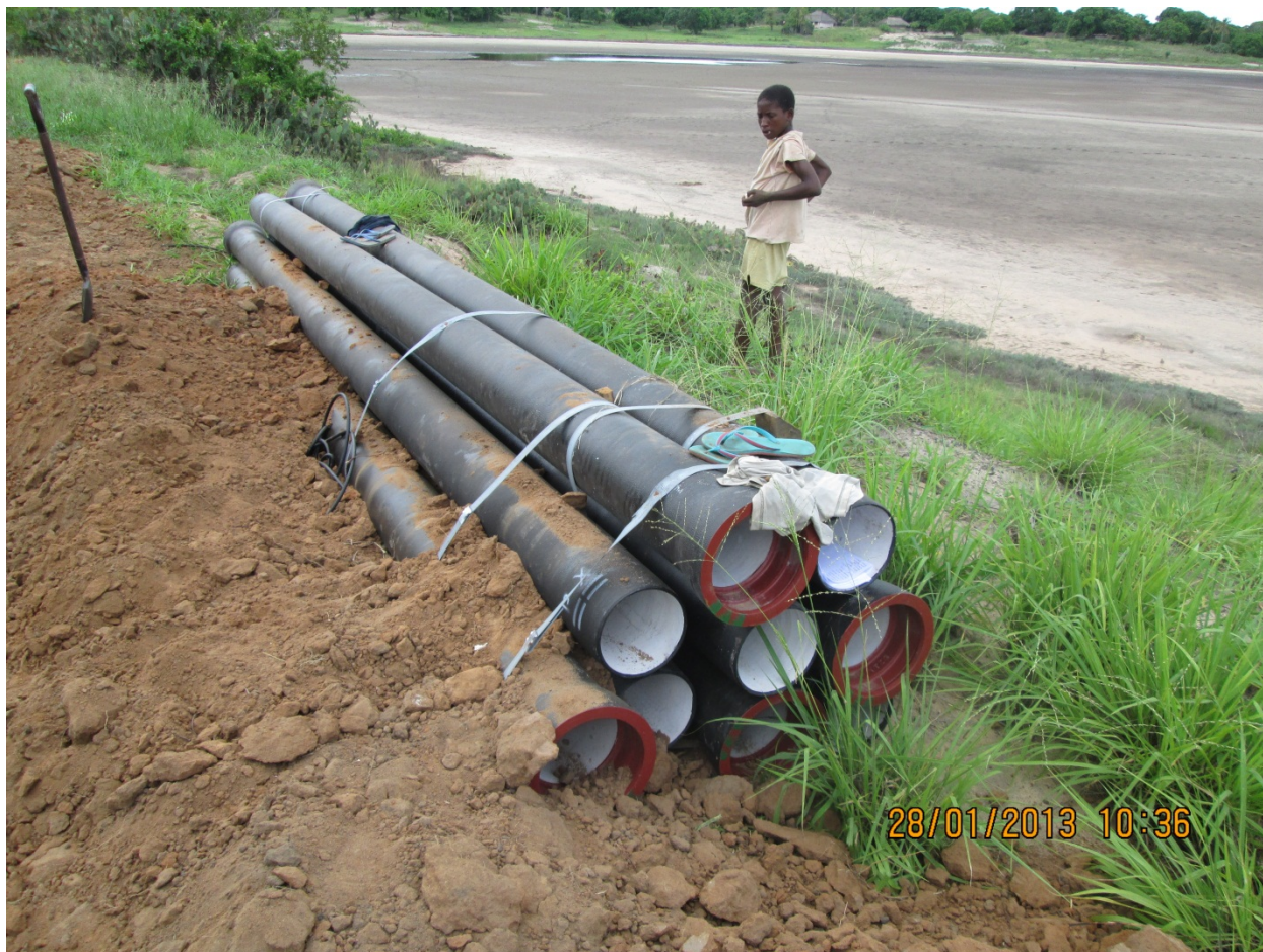
Water supply works
