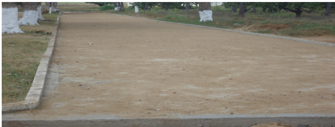
The pavement of the main road in Lumbo Village
