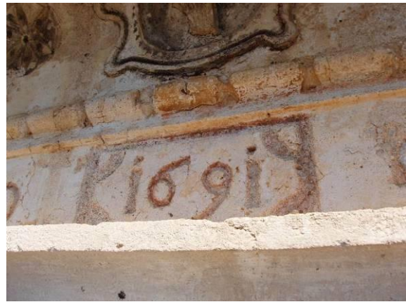
Šestokrilović Palace – Title with year of the construction
