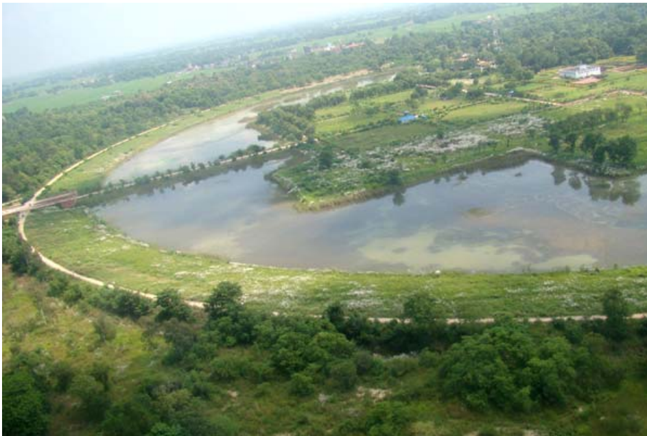
Brick paving of road along circular levee
