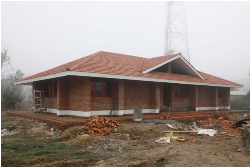
Archaeology building (under completion)
