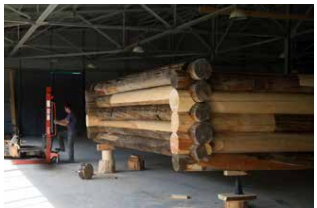
The test-assembly of the restored logs
