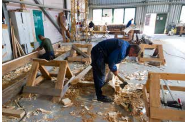
Restoration of logs in the Restoration Complex on Kizhi Island
