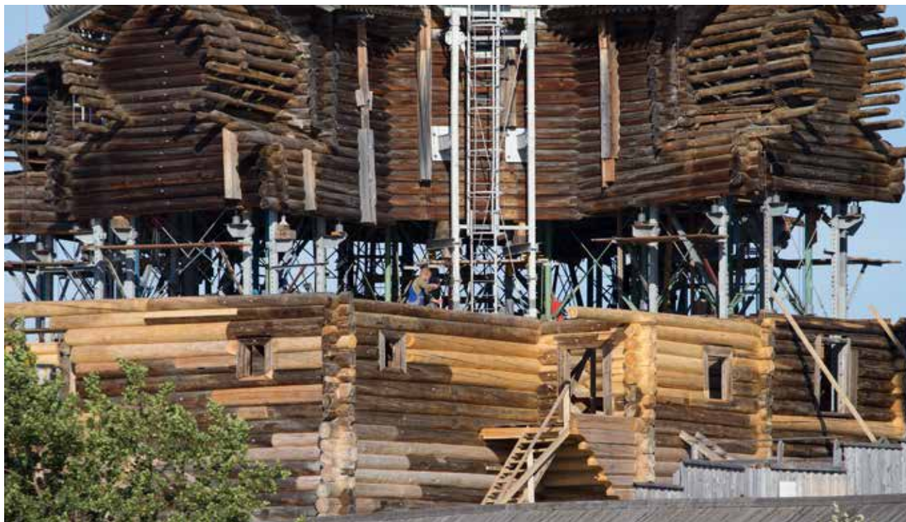
The assembly of logs walls on Pogost
