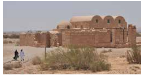
1.4. The main building at Qusayr ‘Amra
