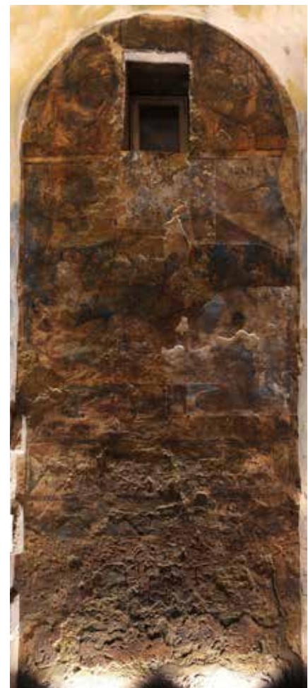
3.17. Raking light photo of South wall, West aisle, showing the plaster's spreading phases
