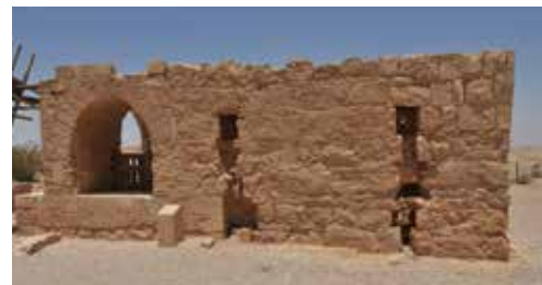
1.5. The saqiya annexed to the main building
