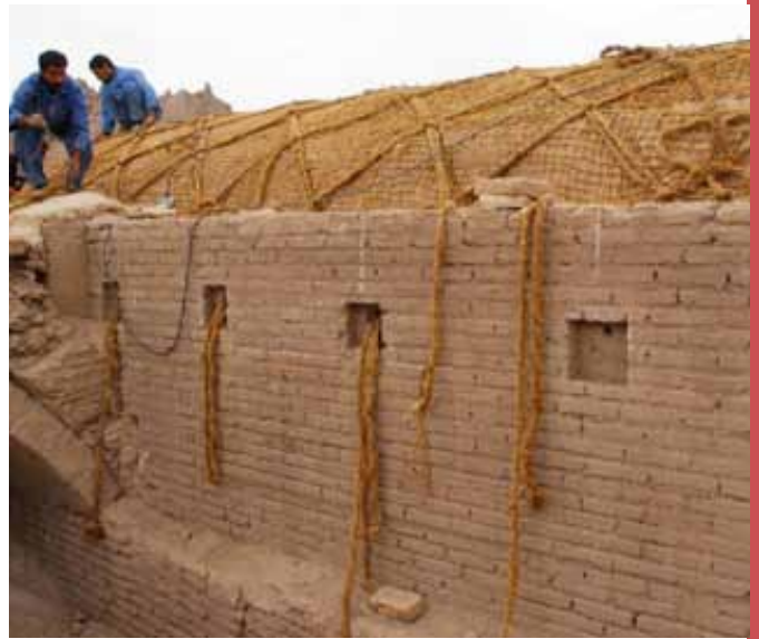
Figure 8: Strengthening an arched roof with rope and mesh made from palm fibre (SIS).
