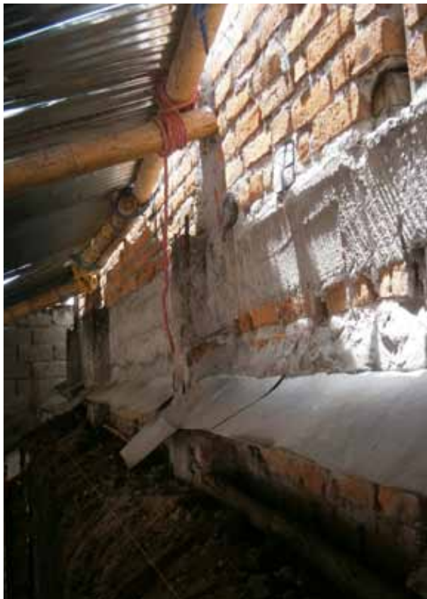
Figure 9: Common wall between the adjoining properties with concrete columns. © María de Lourdes Abad
