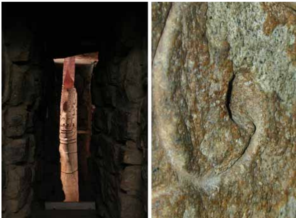
Figure 3: Subterranean channels at Chavín: left, the Rocas gallery in restored condition; right, fractured beams and collapses. © J. Vargas- Neumann
