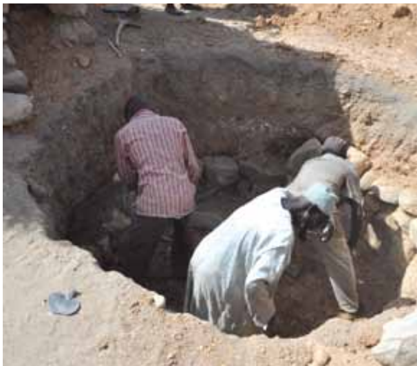
Figure 6: Construction of a sub-basement bullpen. © Michael Thomas
