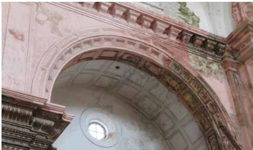
Figure 9: (L) Exposed laterite walls of the Basilica of Bom Jesus showing deterioration of the laterite blocks. (R) Water seepage from the roof affects the wall paintings inside the Church of St Francis of Assisi. © T. Sharma
