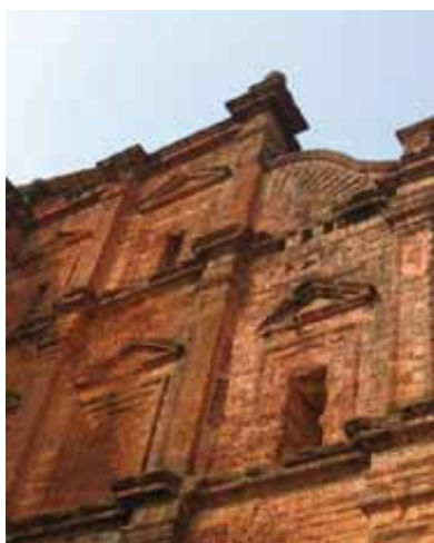
Figure 9: (L) Exposed laterite walls of the Basilica of Bom Jesus showing deterioration of the laterite blocks. (R) Water seepage from the roof affects the wall paintings inside the Church of St Francis of Assisi. © T. Sharma
