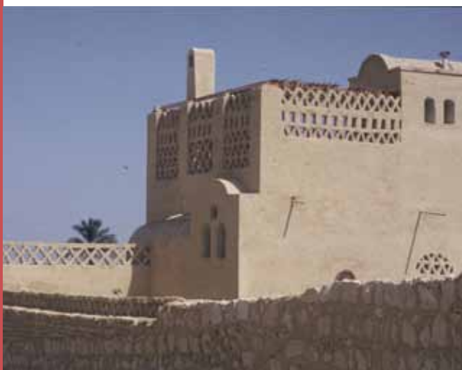
Figure 2: Eco-lodge prototype 'G' for Mr AbdAllah Schleifer, Tunness, Fayoum oasis. Egypt. 1992-93. The mass is intensified by giving the blind walls their due, versus the perforated screening or crowning walls. © AHMAD HAMID ARCHITECTS
