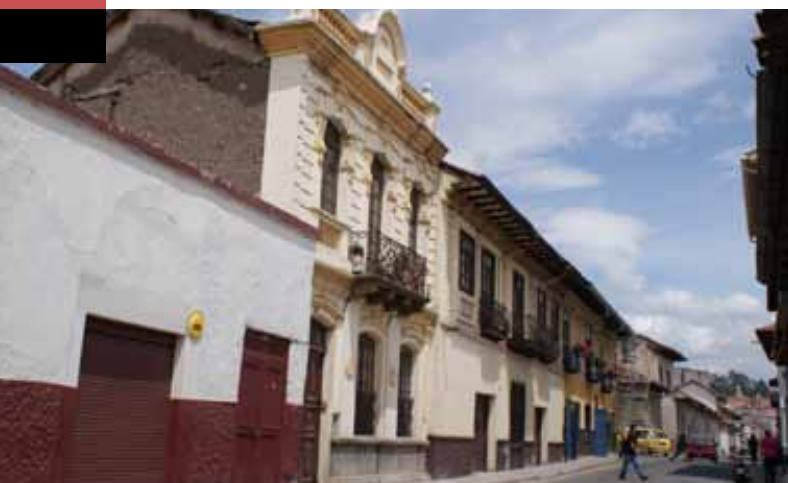
Figure 4: House with brick façade, and interior walls of adobe and wattle and daub. © María de Lourdes Abad
