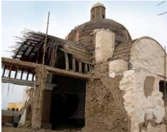
Figure 5: Avoid reinforcements based on beams and reinforced concrete columns, as their different behaviour in earthquake conditions can lead to collapse rather than protect the adobe walls. Damage to the San Luis de Cañete Church in the Pisco earthquake of 2007. © J. Vargas-Neumann
