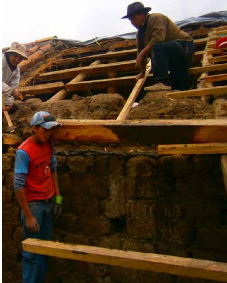
Figure 10: Tile roof with wood, bamboo and mud support structure. © María de Lourdes Abad
