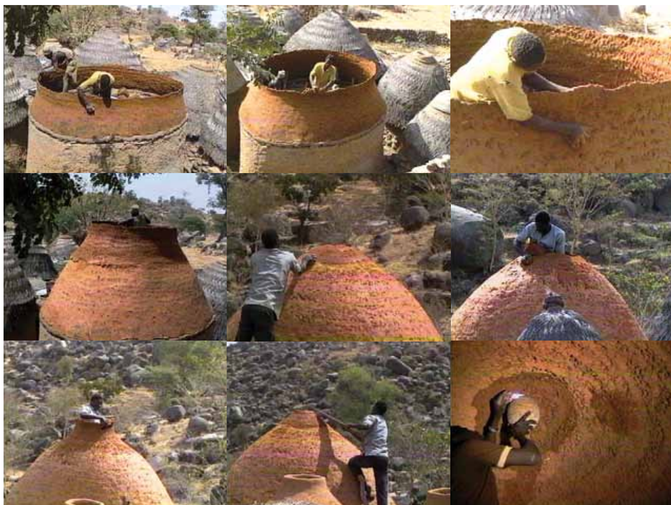
Figure 5: Construction of a Sakun vaulted ceiling, or huruk . © David, 2010
