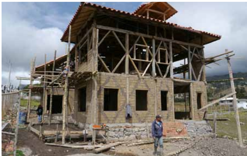
Figure 11: Second wattle and daub house in Cañar, with a structure of recycled eucalyptus poles, bamboo canes and mud filled with compressed earth blocks. © María de Lourdes Abad
