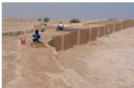
Figure 12: The inner wall before and after restoration. © M. H. Talebian
