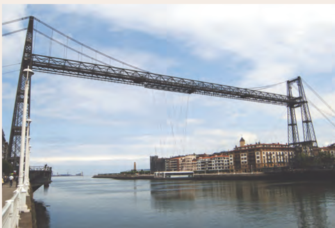
Vizcaya Bridge (Spain)
