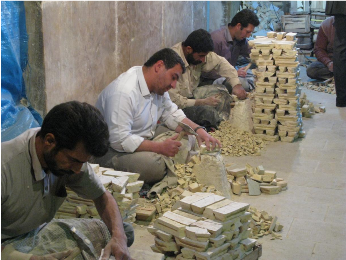
Figure 19. Royal Mosque Dome tile restoration workshop
