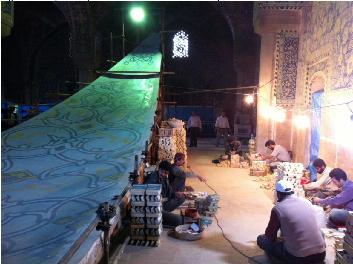
Figure 18. Royal Mosque Dome tile restoration workshop
