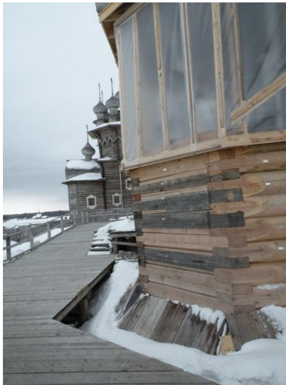
Figure 10 7th tier logs reinstated in the building. April 2013
