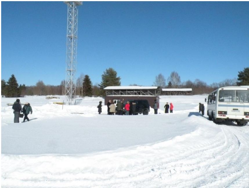
Figure 8 Infrastructure – log storage & telecommunications. April 2013
