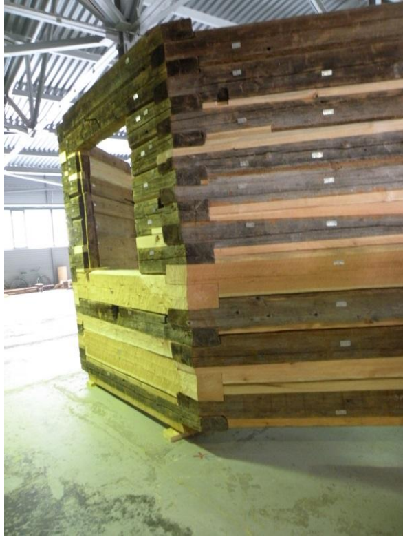
Figure 11 6 th tier logs reassembled and repaired in the workshop. April 2013.
