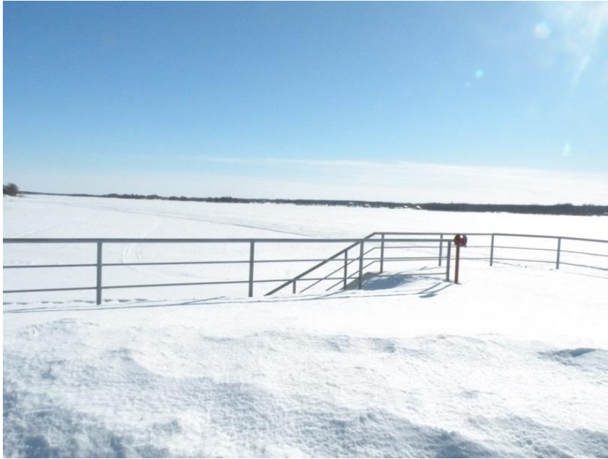
Figure 7 The new wharf completed 2011. April 2013
