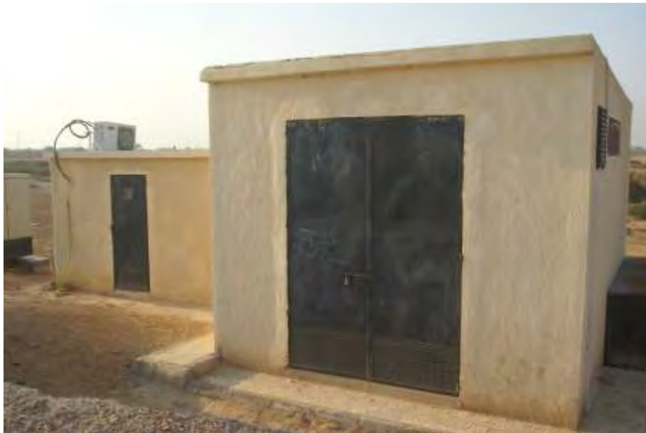
Figure 6. Illuminated access road leading to main basilica and one of several dewatering pump service buildings located along its length
