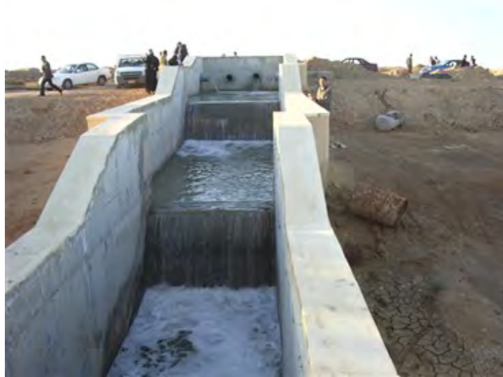
Figure 5 One of the weirs discharging the drained water after two hours of pumping. The rate of flow is of the order of 0.05 \text{ m}^3/\text{s}
