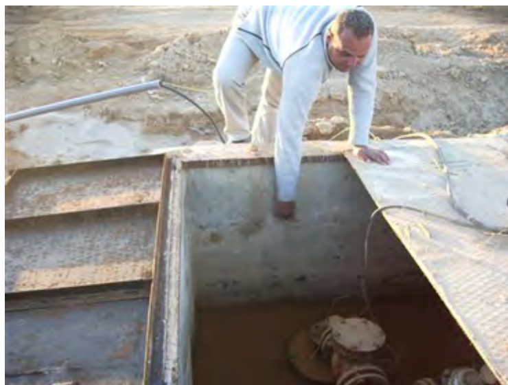
Figure 6 An attendant shows how the water level has lowered after two hours of pumping
