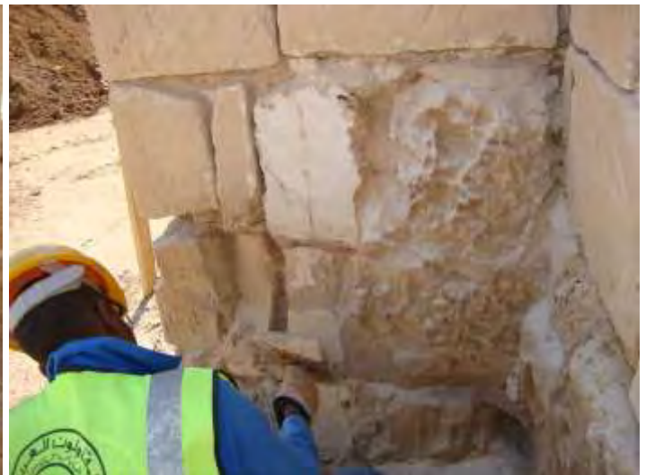
Re-facing of original blocks to new elevation
