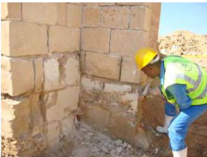
Figure 13. Replacement wall. Retained original refaced blocks can be identified as slightly darker in colour. Presumably the new stone is from a different source to the original.
