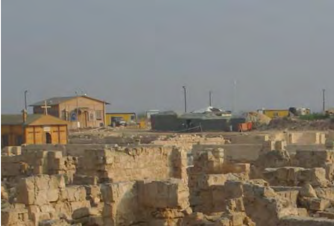
Figure 7. Construction of structures at the main basilica
