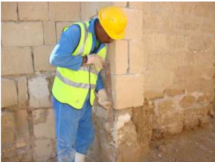
Determining new elevation for wall
