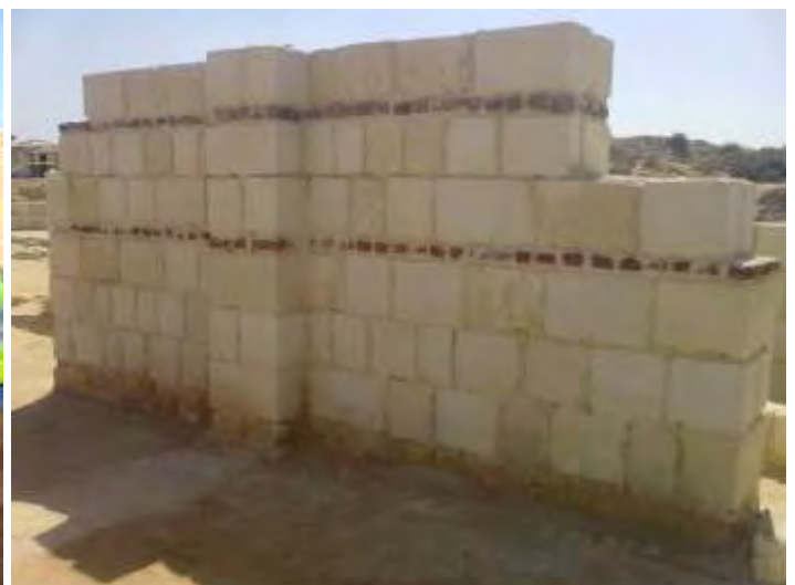
Figure 13. Replacement wall. Retained original refaced blocks can be identified as slightly darker in colour. Presumably the new stone is from a different source to the original.
