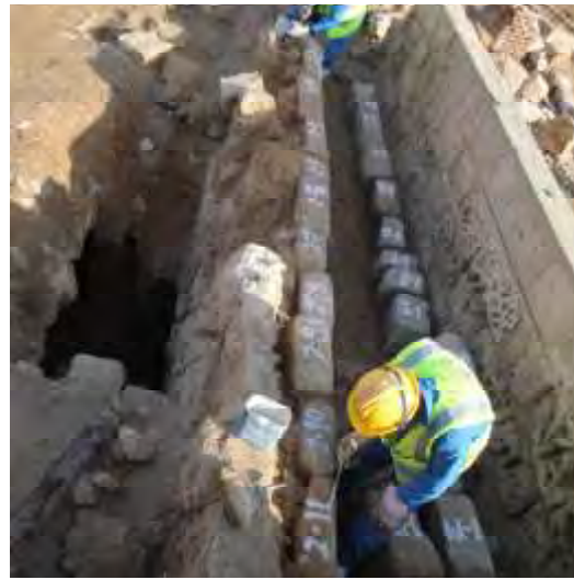
Dismantling an original wall
