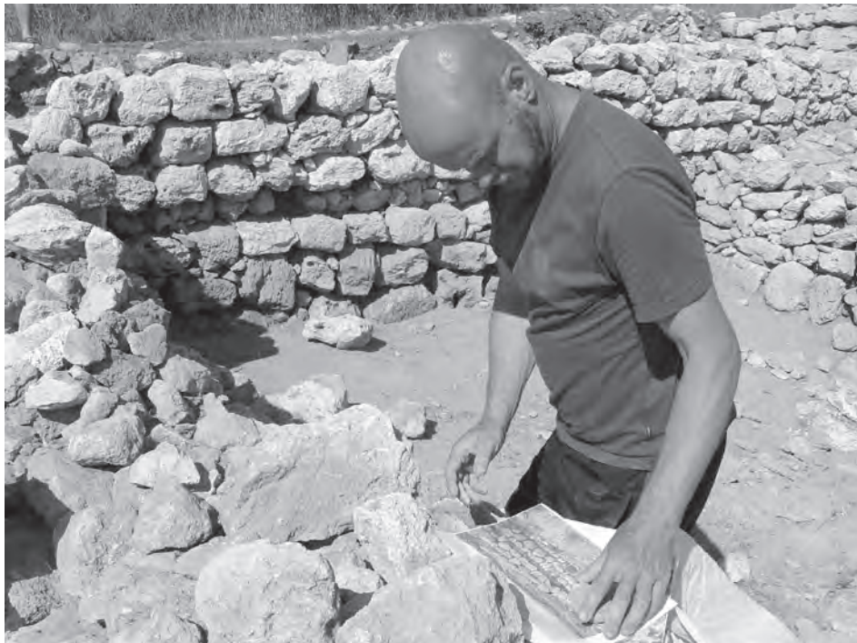
Figure 8. Conservator Jonathan Kemp uses a print-out of a detailed wall face photograph to help reconstruct a section of collapsed wall, 2004.
