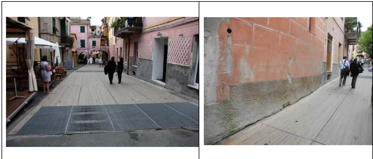
Figures 13 and 14. New movable wooden slabs and grills in Monterosso streets
