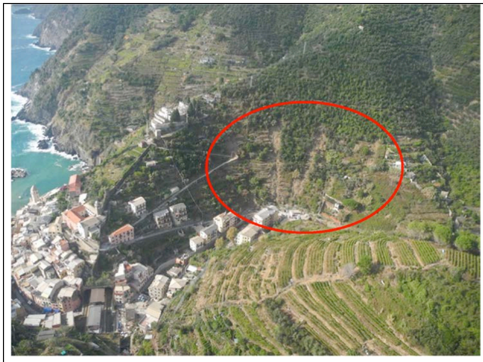
Figure 15. Landslides in Vernazza surroundings, October 2012
