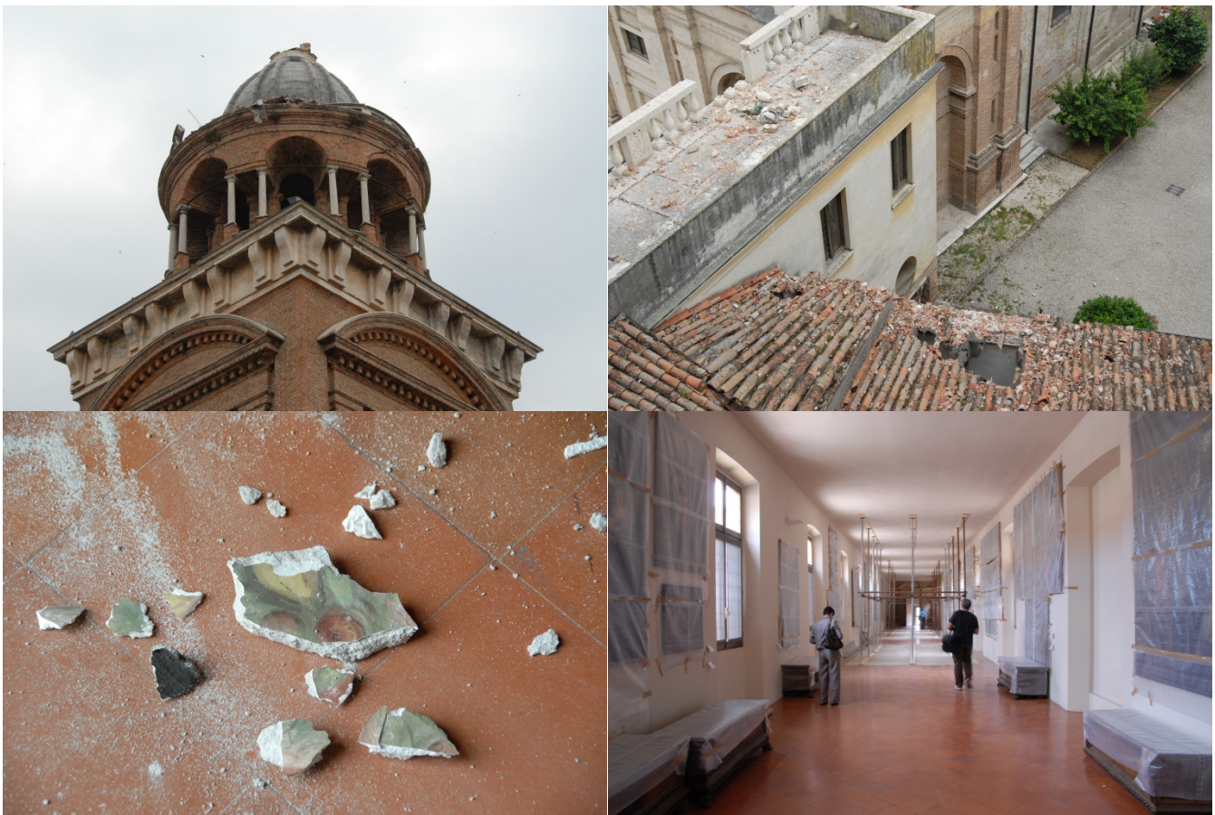
Figure 17 – Above, the collapsed turret of the bell-tower, Church of Santa Barbara (Palazzo Ducale, Mantua). Below, fallen fragments of painted decoration (left) and safety measures within the galleries of the Museum (right).
