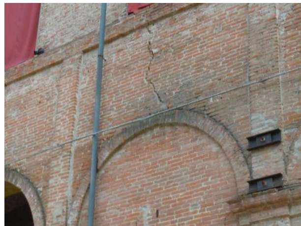
Figure 12 - Left: the disassembled roof of the collapsed turret of Palazzo Paradiso, in Ferrara. Right: cracks on the façade of Palazzo Massari, which houses the civic modern and contemporary art gallery.
