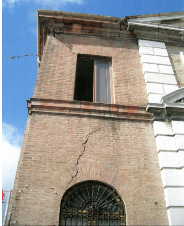
Figure 13 - Left: cracks on a southern bastion of the City Walls; right: cracks on Porta Paola
