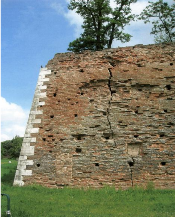
Figure 13 - Left: cracks on a southern bastion of the City Walls; right: cracks on Porta Paola
