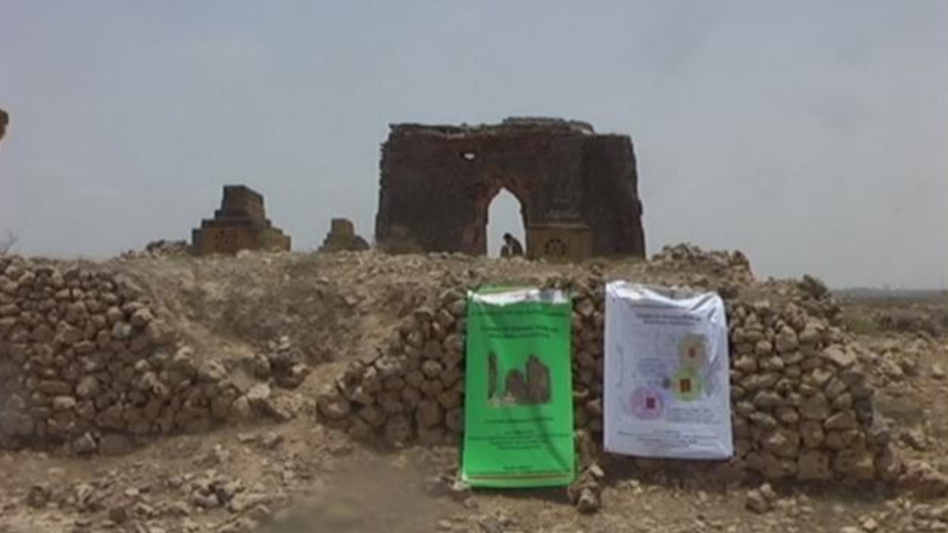
120510 Consolidation project Heritage Foundation
