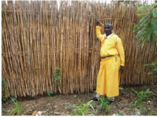
Detail of the new emergency reed and steel fence.
