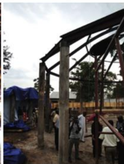
The main structure of RC columns and curved steel beams. The Mission noted concern about the shallow roof incline.
