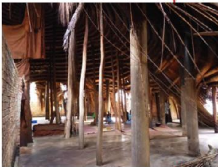
The interior in Nov 2010. Note RC columns and timber columns as at Kasubi.
