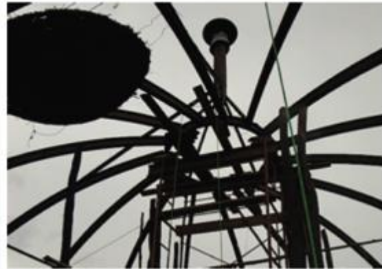
The repaired steel structure – the new ceiling will hang from the structure. Note the portion of the old ceiling that remains on site during the repair and maintenance works.
