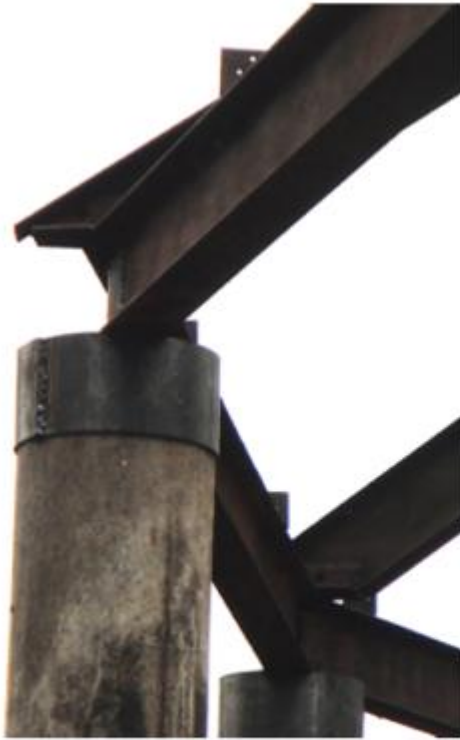
The new steel caps and beam connection.
