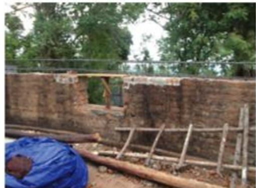
The state of new works on the outer wall: Reinforcement for the new RC ring beam.
