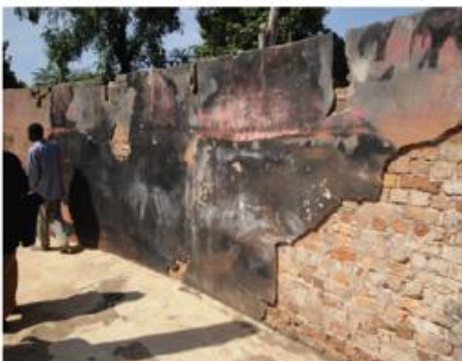
The outer wall of the tombs showing the condition of the cement plaster – note the structure had no RC ring beam.
