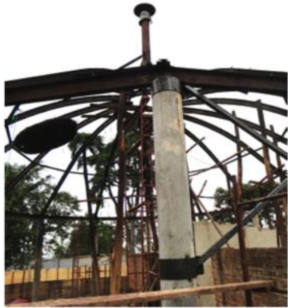
The complete steel roof structure – the temporary cross bracing between RC columns is to be removed as soon as the roof bracing has been fitted.
