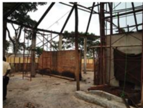
The RC columns have received steel caps. The steel roof elements have been straightened and refitted.
