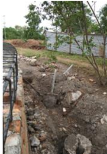
Preparing for the new outer columns.
