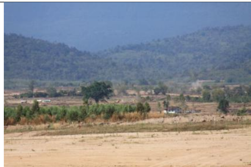
Figure V.3: Construction site of Huay Samong Dam
