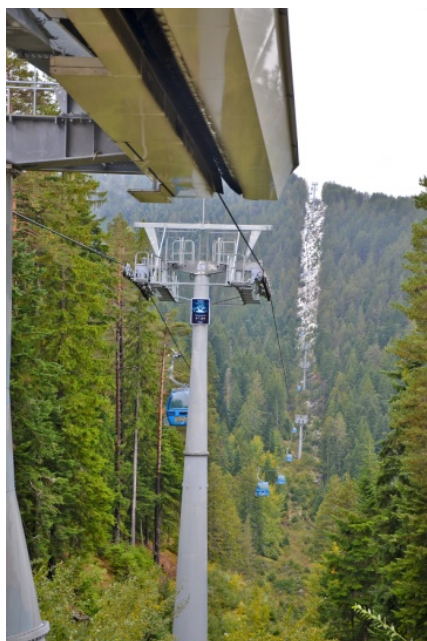
Photo 5. Clearing of the gondola lift.
