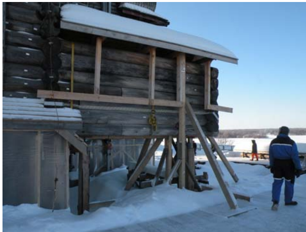
Figure 3 – Temporary bracing at the Church of the Transfiguration.
