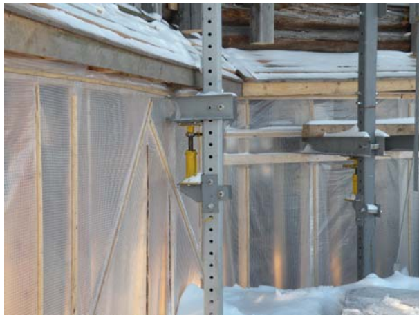
Figure 2 – Lifting set-up at the Church of the Transfiguration
