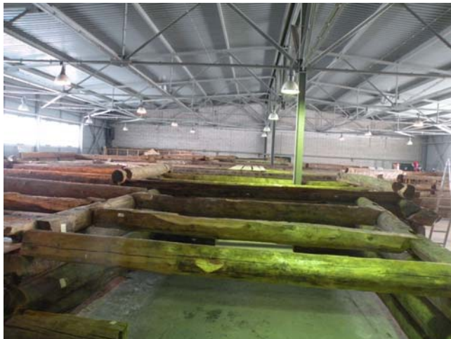
Figure 6 – The 7 th tier of logs reassembled for analysis and repair.
