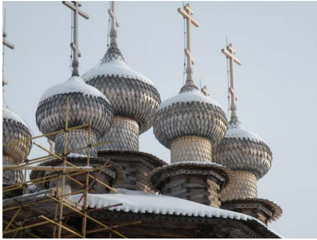
Figure 8 – Newly repaired domes on the Church of the Intercession.
