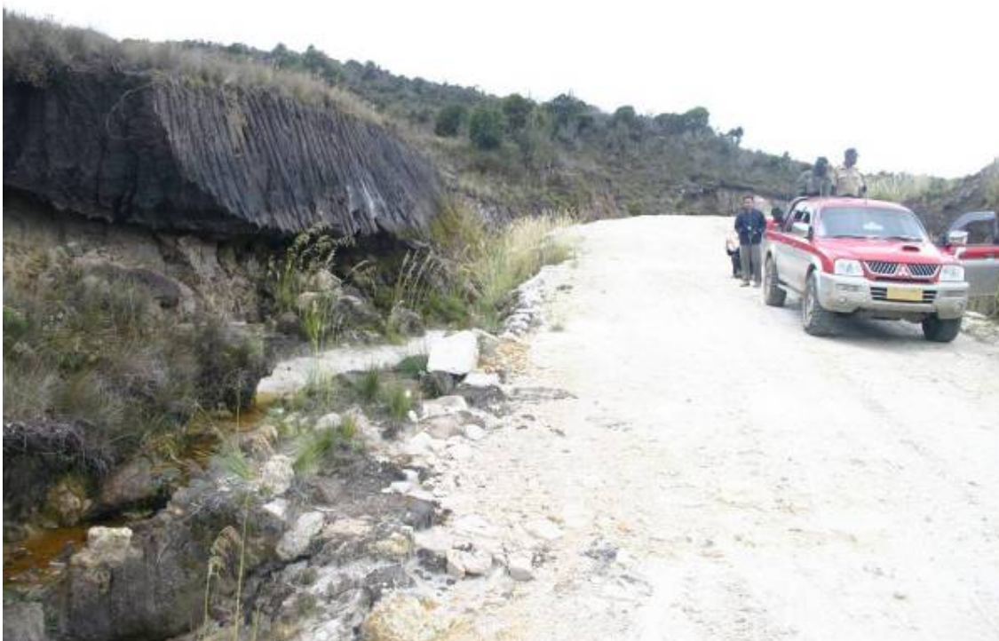
Photo 13: Construction of Habema-Nduga-Kenyem road through fragile peat bog.
