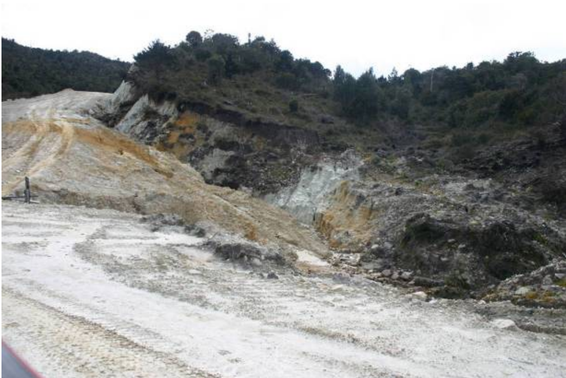
Photo 17: Extensive erosion on Habema-Nduga-Kenyem road.
