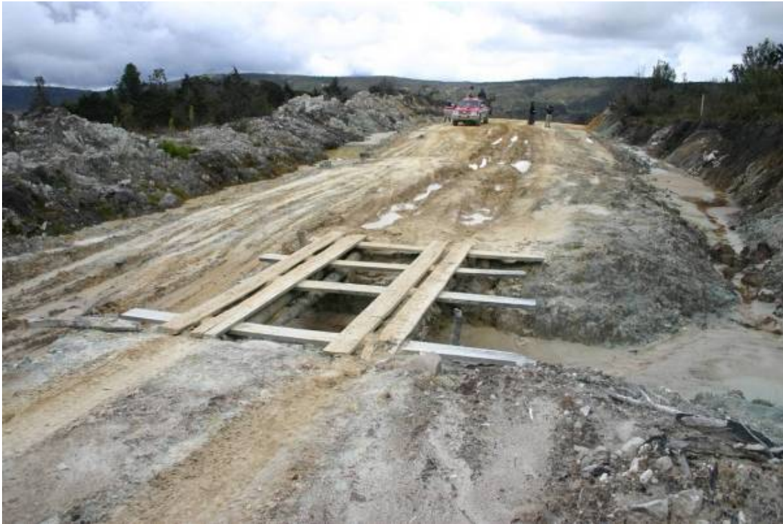
Photo 14: Temporary bridging and extensive erosion on Habema-Nduga-Kenyem road.
