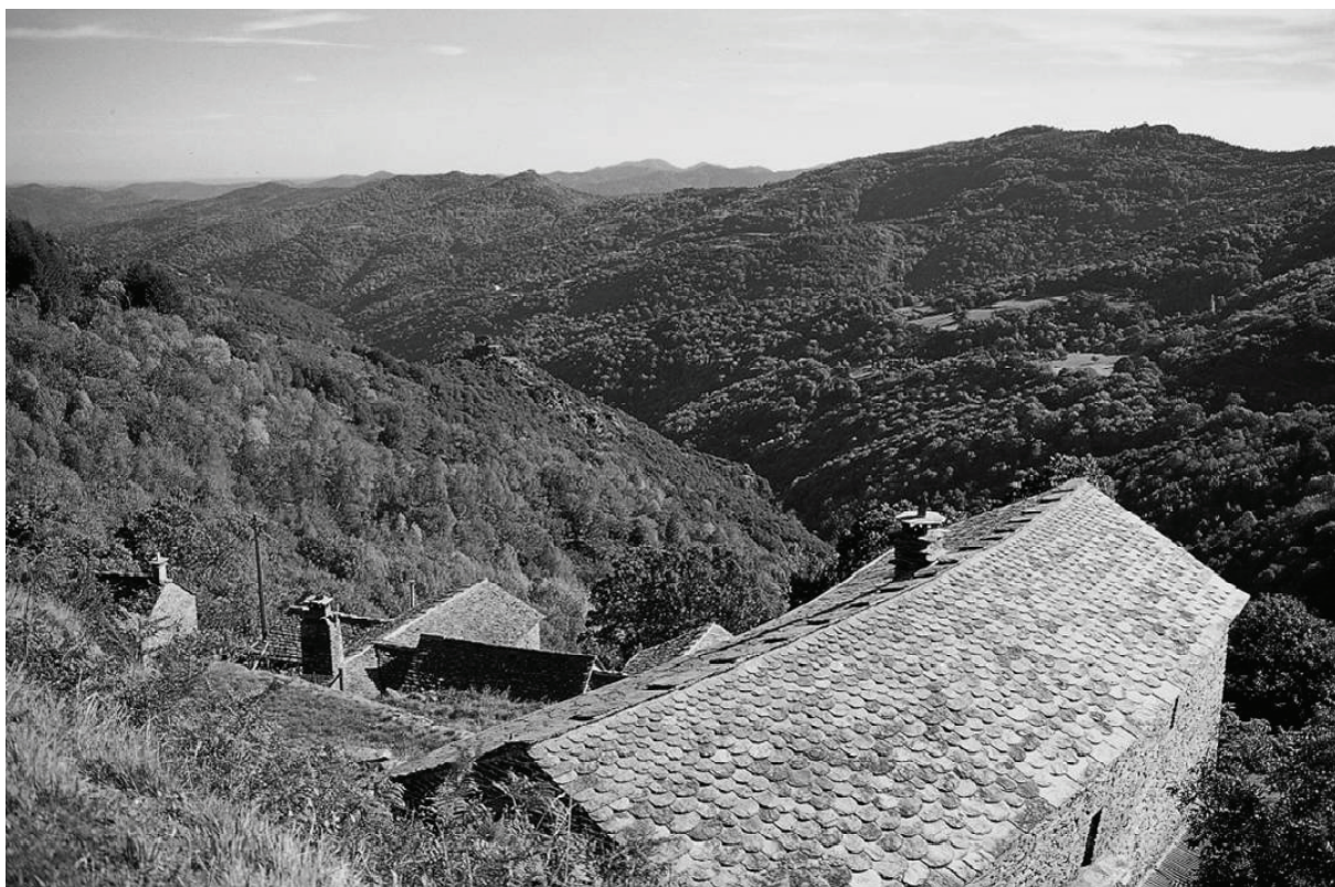
Roof in shell-shaped slates
