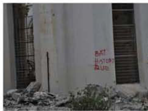
ISPAN identified and marked all buildings of heritage value
