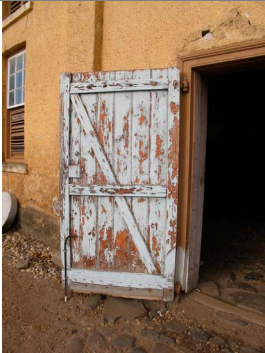
Original ledged, braced and sheeted door (D01)
