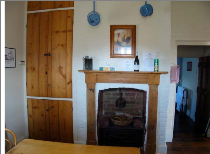
Space G01 showing original timber chimneypiece and built in cupboards.
