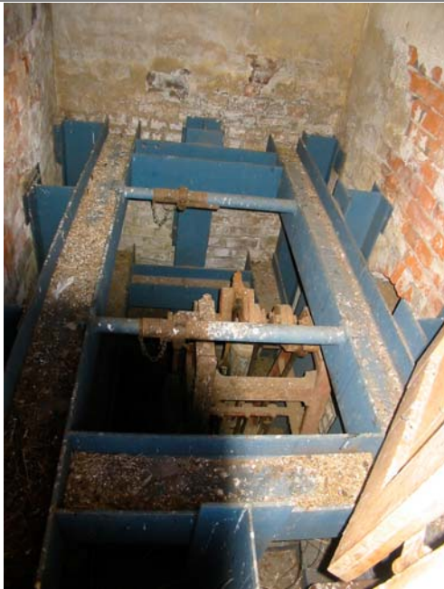
Adjustable metal structure support in Pump Room (Space G02)
