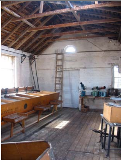
Space G01, showing exposed timber roof framing and 1920s apple grader on left.
