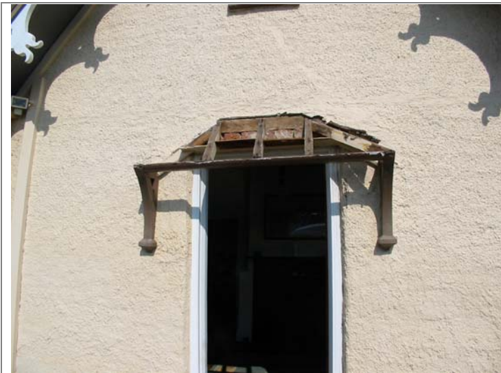
Detail of timber hood to front door (D01) on east elevation
