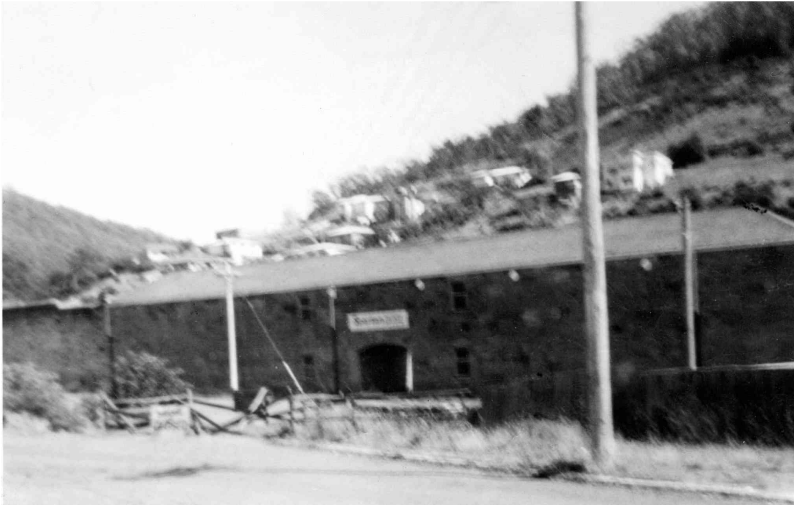
Figure 14 Wall to Yard 3 on Degraeves Street (south side), c. 1947. Source: Cascades Female Factory Historic Site Pty Ltd.
