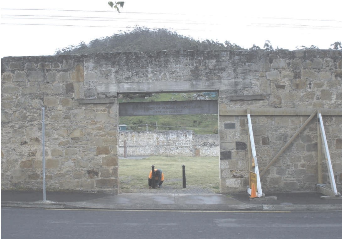
Figure 4 Entrance to Yard 1, Degraeves Street (south elevation).
