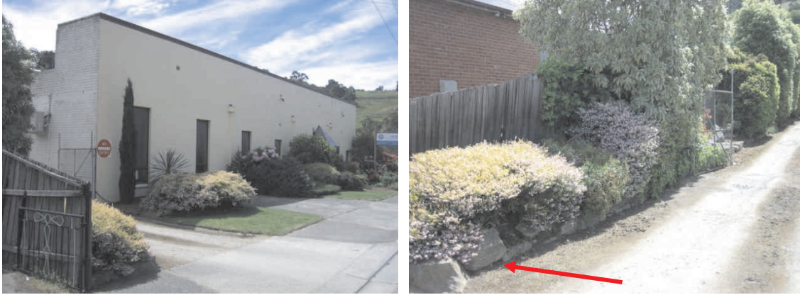
Figure 20 Current views of the church building and the western driveway boundary of the church property. Note the in situ sandstone wall footing running the length of the driveway.
