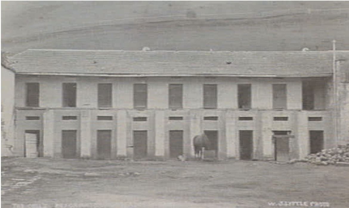
Figure 11 'The Cells, Reformatory, Cascades, Hobart' undated. Note horse in centre picture, and demolition underway. Source: State Library of Victoria picture collection (Image No. a09418).
