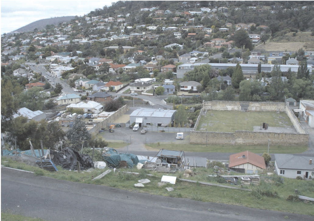
Figure 2 Elements of the former Cascades Female Factory, viewed from the north, with (from left to right) Yards 4, 3 (centre picture) and 1.
