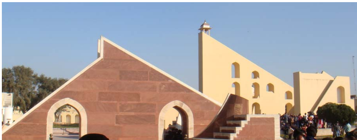
Fig. 4: Lime plastered Brihat Samrat Yantra behind the sandstone clad structure in front
