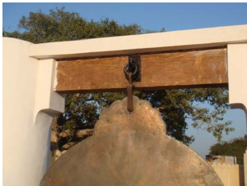
Fig.8: The Yantra Raj with replaced wooden beam
