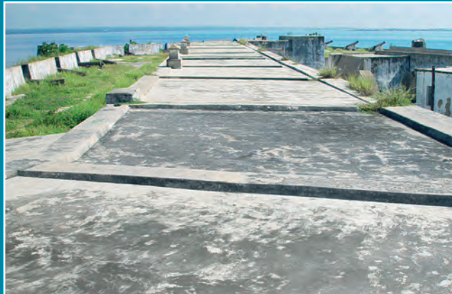
Coral stone roof slab reconstruction and waterproofing.
