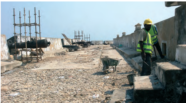
Removal of intrusive vegetation and NW terreplein surface reconstruction.
