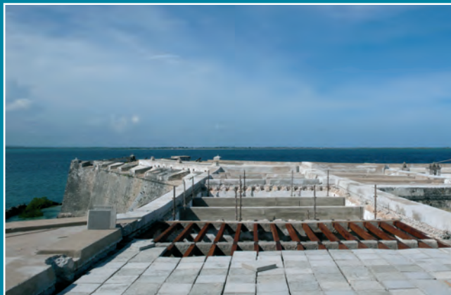
Coral stone roof slab reconstruction and waterproofing.
