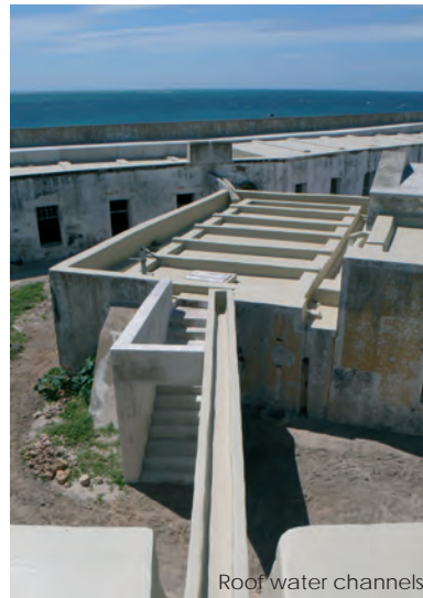
Roof water channels
