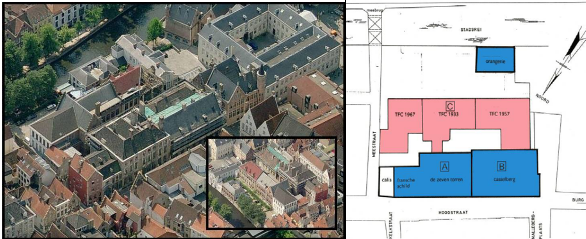
The telephone exchange building complex near the Hoogstraat (Source: City)
