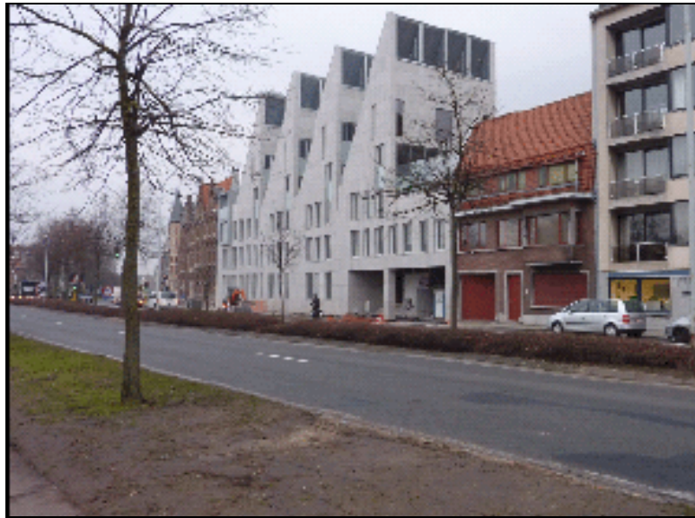
Apartment project realisation "Gulden Vlieslaan" (Source: City)
