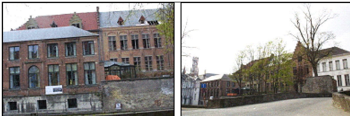
Demolition of centre plot buildings on the former telephone exchange area which are considered by the city services and Flemish authorities as an obstacle to the recovery of the historic complex (Source: City)
