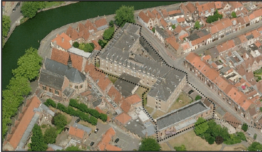
The current buildings erected in 1972, will be demolished. On this site a new old people's home will be built. (Source: City)
