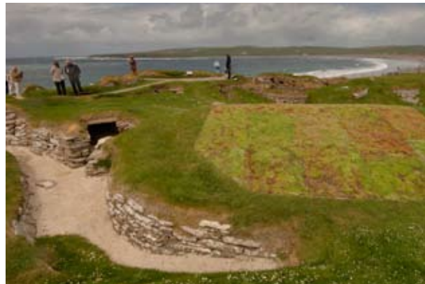
The new roof over Hut 7 at Skara Brae
