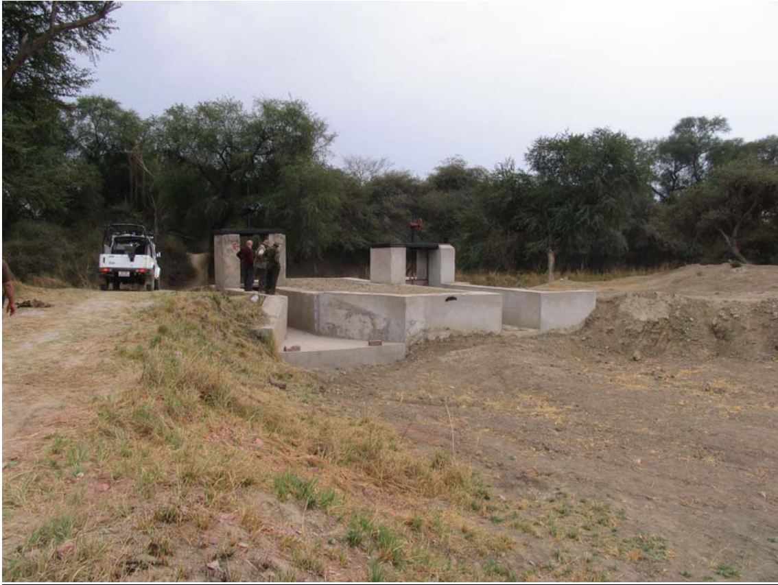
The new water control structure connecting the Chiksana Canal to the Park. Picture by Marc Patry.
