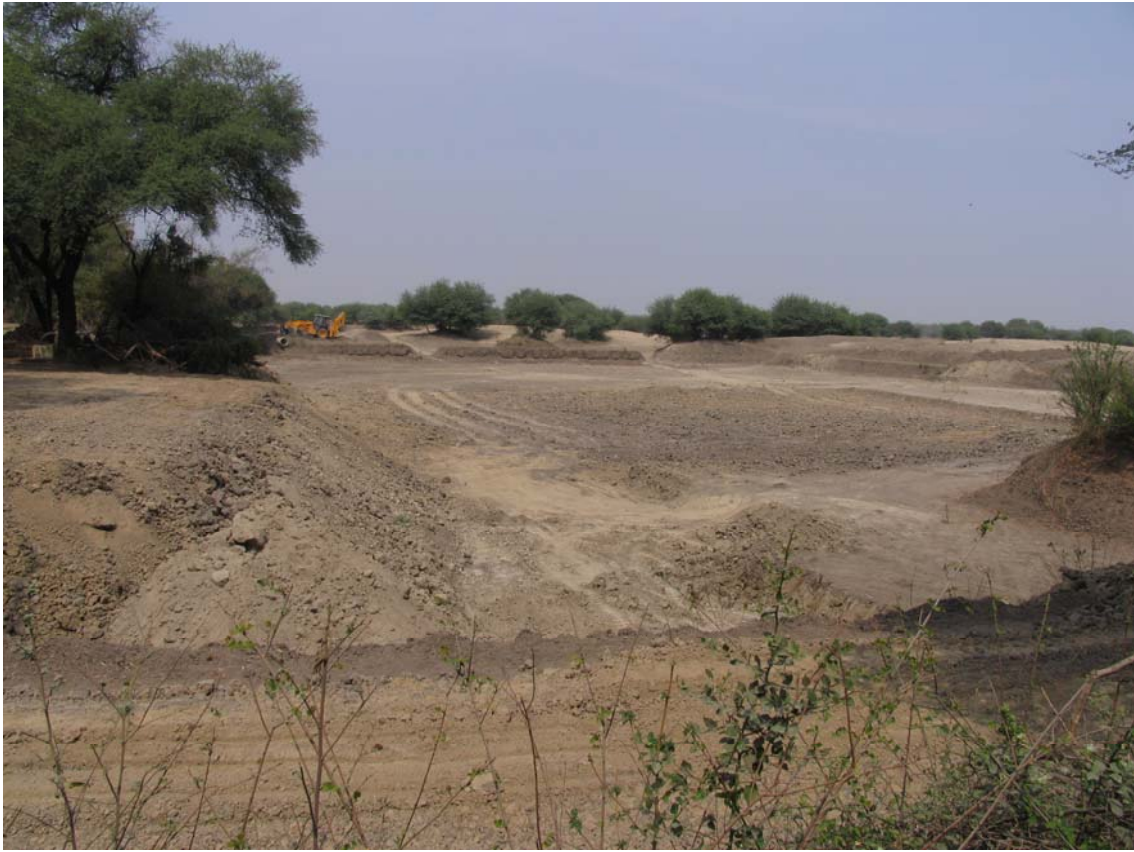
Construction of a new deep pond to retain fish from one monsoon to the next. Picture by Marc Patry.
