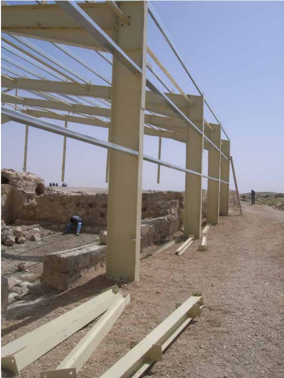
Picture 11 : Load-bearing structure outside the perimeter of the ancient walls
