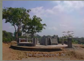
The construction of the office, the laboratory, and store room
