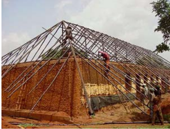
Reconstruction of the roof of the Adjalala
