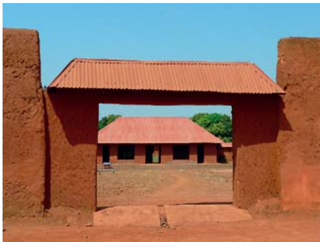
The entry gate after restoration
