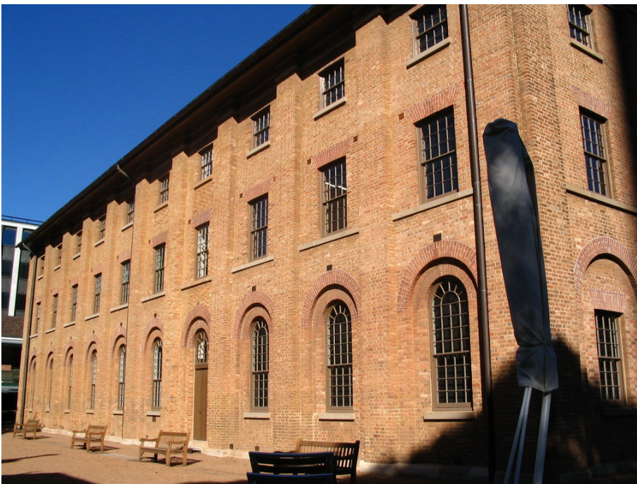
Figure 17: Current condition of the site – detail of façade of and north-facing wall of brick central Barracks building showing state of conservation of exposed brick facades with stone footings (ground level), window treatments and graveled surface of courtyard, all in good to very good condition.
