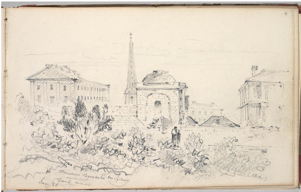
Figure 12: Some of the key components of the site and its setting are shown in this historical sketch from 1835 by Robert Russell: the central dormitory building to the left, and the north-east pavilion or cell in the centre. The southern end of the General, or Rum, Hospital is on the right, and the distant spire of St James' is in the centre. The sketch is probably drawn looking westwards from the Domain, with the vegetable gardens and flogging yard hidden by shrubbery in the foreground.
