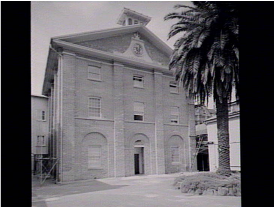
Figure 10: View of Hyde Park Barracks during first phase of works to remove Court structures and convert to a museum use in 1976. Source:
