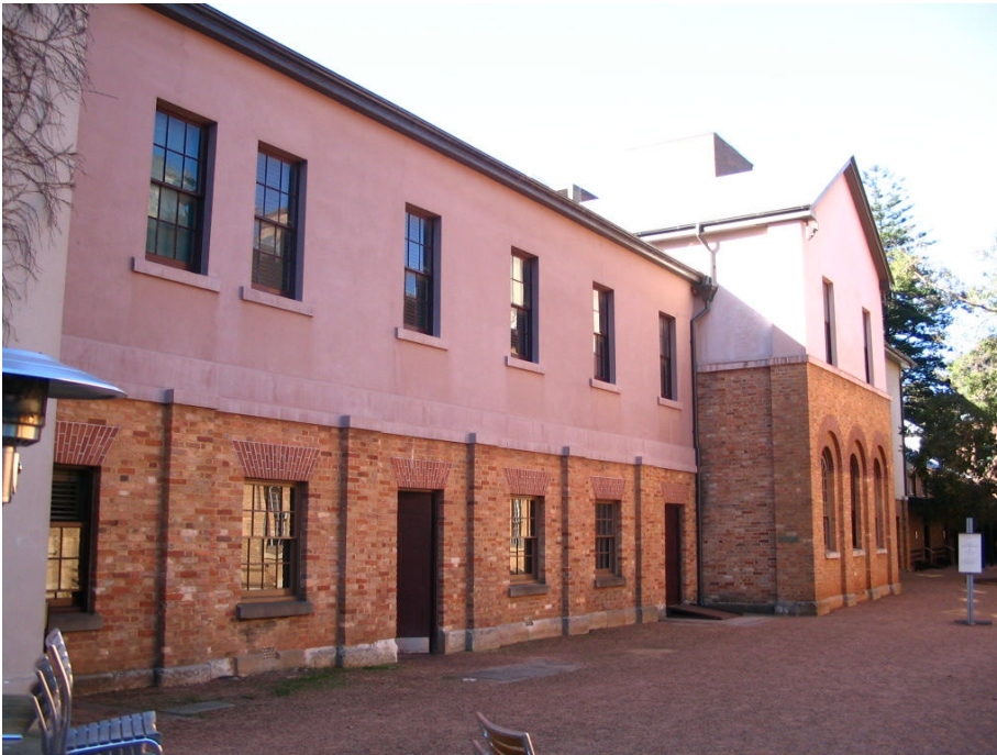
Figure 16: Current condition of the site – detail of façade of brick northern range of buildings showing state of conservation of exposed brick facades with stone footings (ground level) and rendered brick (upper level), window treatments and graveled surface of courtyard, all in good to very good condition.
