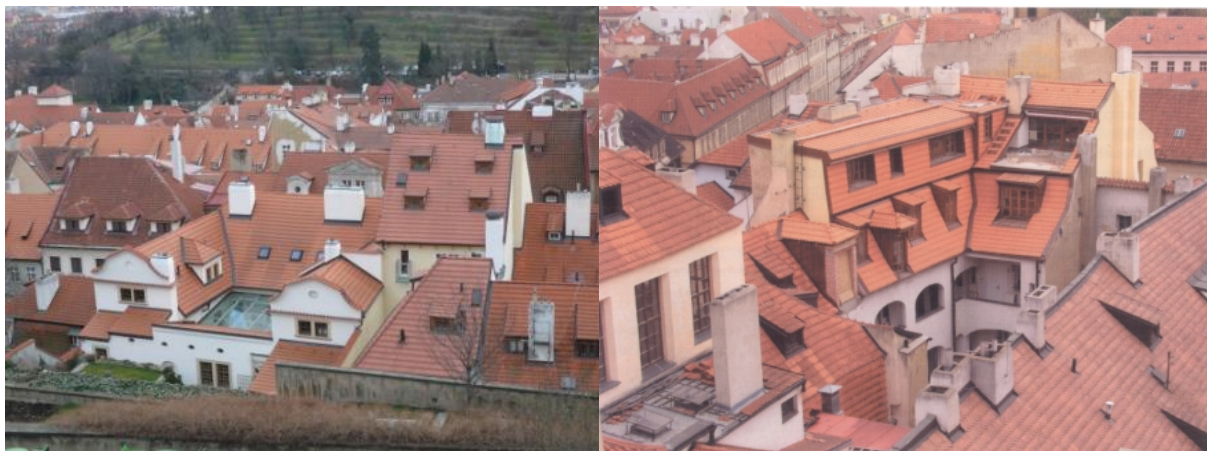
Examples of transformation of roofs in the historic centre
