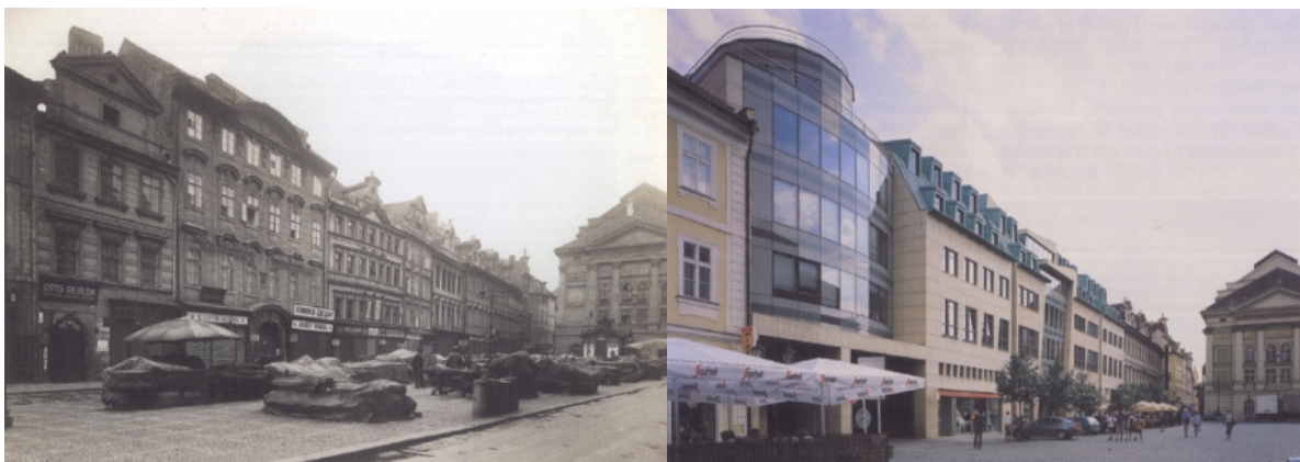
Buildings in Ovocný Square, demolished in 1929, and new constructions of the 1990's on the same site
