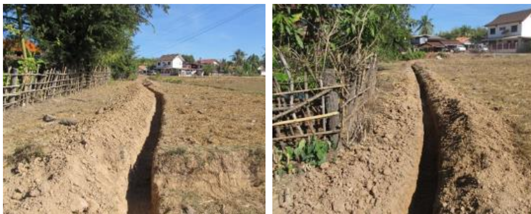
Figure 6 Completed excavation of the new channel for water pipeline.
