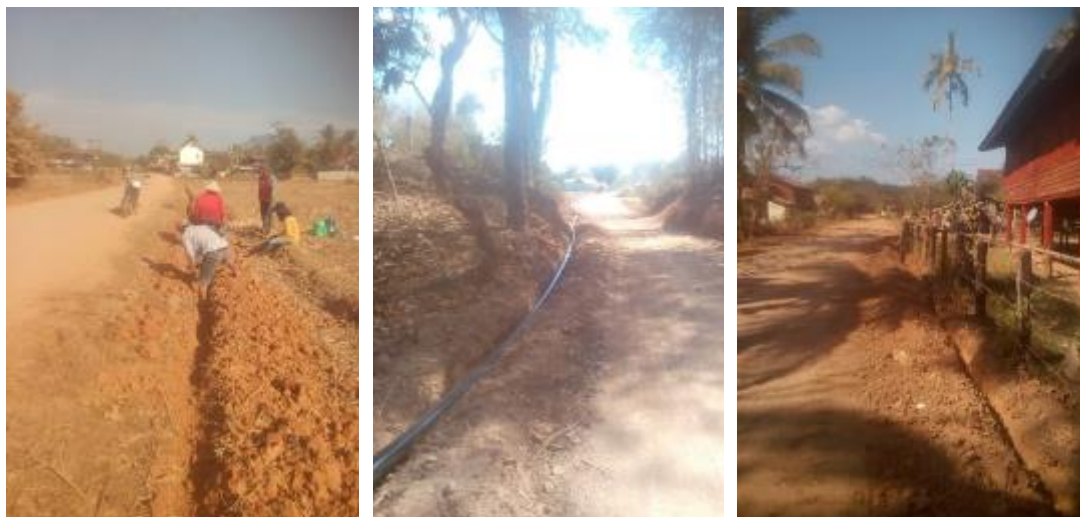
Figure 7 Pipeline installing on the area inner ancient wall and Phanone village.
