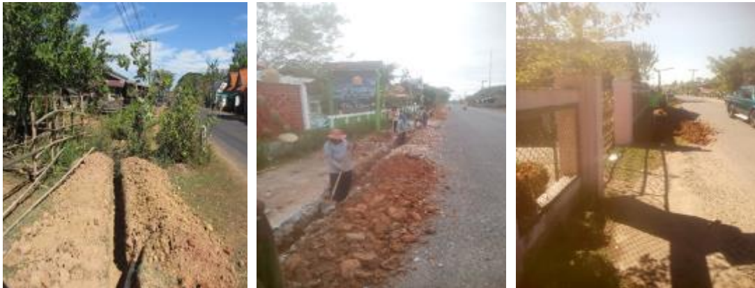
Figure 10 Pipeline installing from Vat That village to Houy Phabang Bridge (digging two lines)
