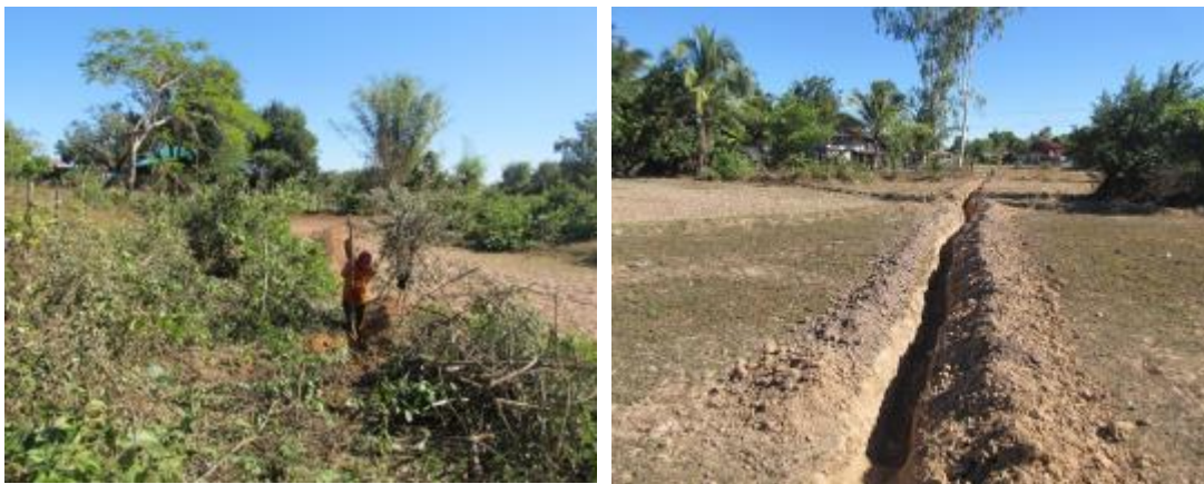
Figure 5 The channel's line has been changed from the remain to farmland area to avoid impact to the properties.
