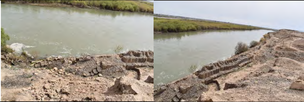
Current status of gabion protection of the eastern Tell © ICOMOS/Y.Makaroun
