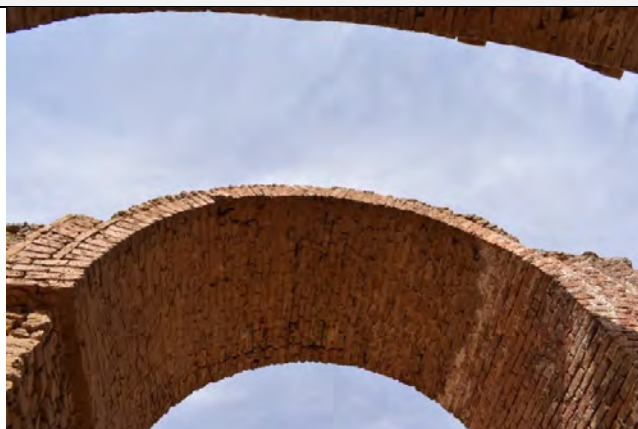
View of the middle arch intrados with some cracks and unstable elements ©ICOMOS/Y.Makaroun 2022
