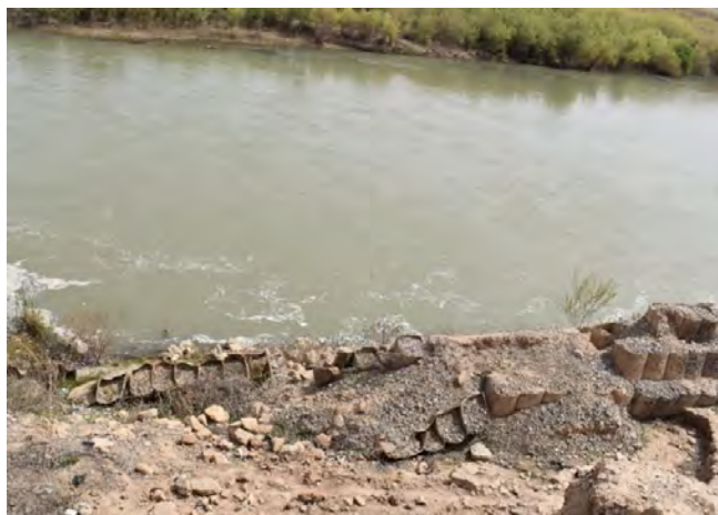
Figure 8 – Damaged riverbank protection measures © ICOMOS/Y.Makaroun
