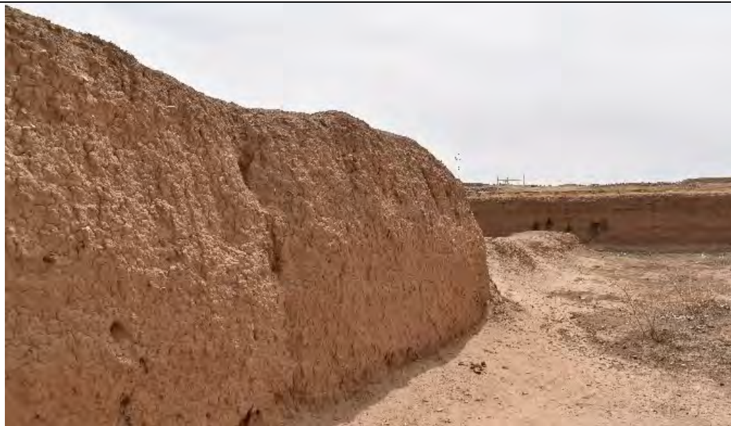
Eroded vertical walls © ICOMOS/Y.Makaroun
