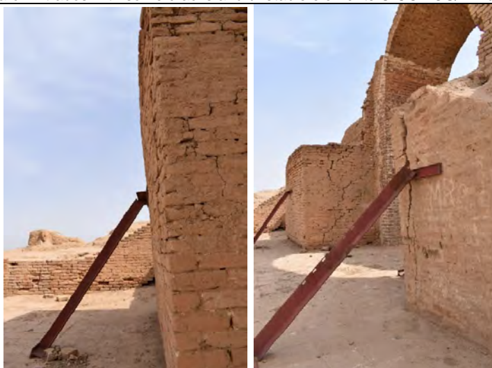
Detailed views of propping system on the outer elevation of the gate © ICOMOS/Y.Makaroun
