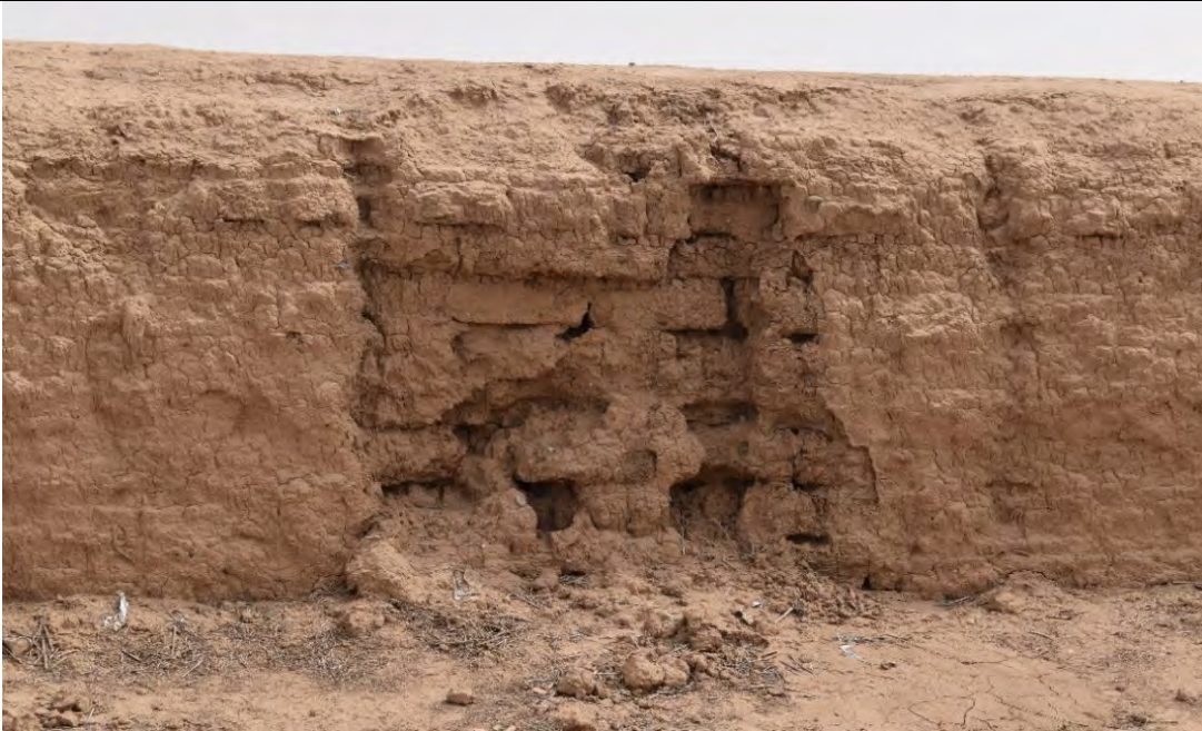
Detail of typical decay process and sun-dried mud brick masonry © ICOMOS/Y.Makaroun
