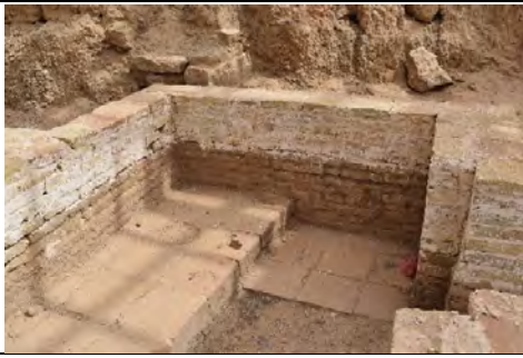
Details of reconstructed baked brick masonry © ICOMOS/Y.Makaroun
