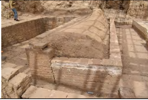
Details of reconstructed baked brick masonry © ICOMOS/Y.Makaroun
