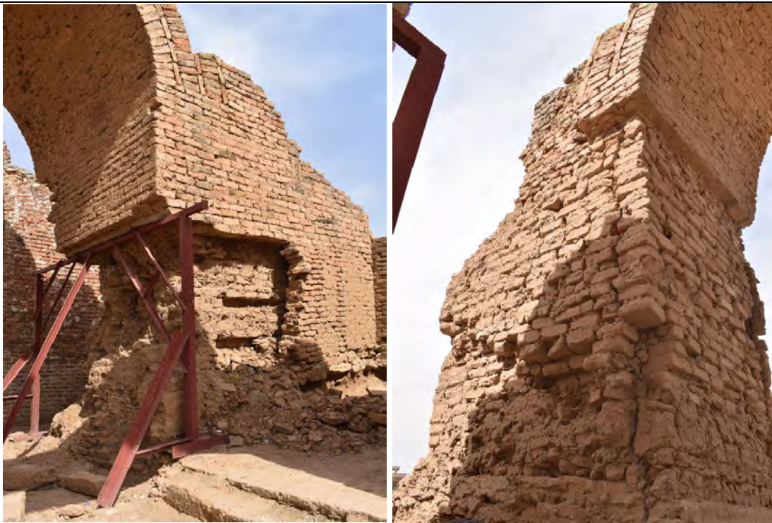
Details of propping and surfaces cleaned © ICOMOS/Y.Makaroun
