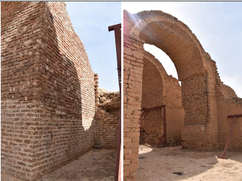
View of the outer arch pile restored with new baked brick and propping © ICOMOS/Y.Makaroun
