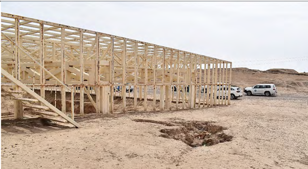
Western side of the shelter with deep erosion of the ground © ICOMOS/Y.Makaroun
