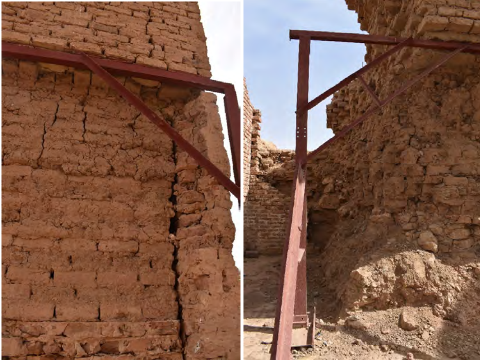
Views of middle arch propping system and cracks (©ICOMOS/Y.Makaroun 2022)
