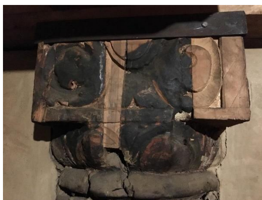
Figure 21 - High-quality modern repair from elsewhere in Jokhang Temple, 10 April 2019.
