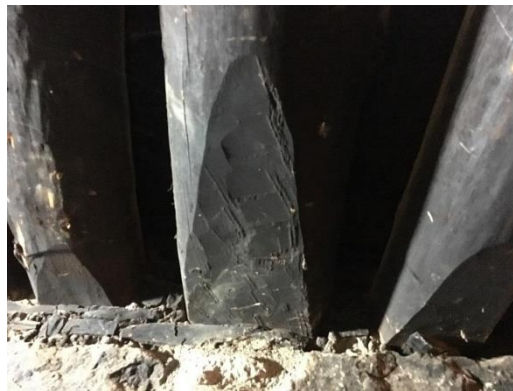
Figure 19 - Adzed joist ends in the foundations of the Potala Palace exhibiting tool markings (witness marks) that match the carpentry tools depicted in the mural at Norbulingka Palace, these being typically narrow width adzes hafted on long handles, 12 April 2019.
