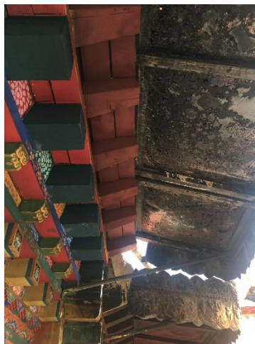
Figure 8 - Fire damage to the roofing at the eaves of the second-floor mezzanine, immediately below the parapet wall, 10 April 2019. Note the unfinished gilding.
