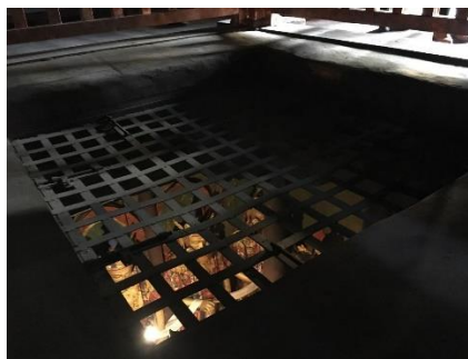
Figure 15 – The original, screened inlet remains in place, 10 April 2019.
