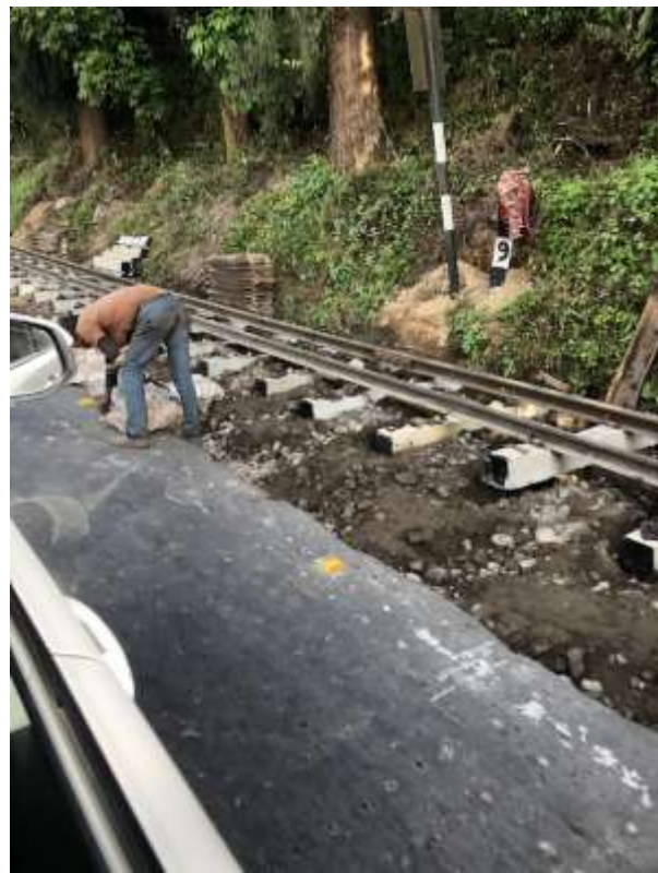
Relaying tracks on concrete sleepers, DHR © M. Pearson 2019
