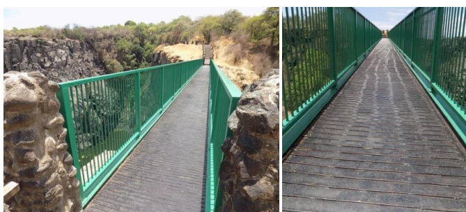
Newly refurbished floor and barriers of the Knife-Edge Bridge in the Victoria Falls
