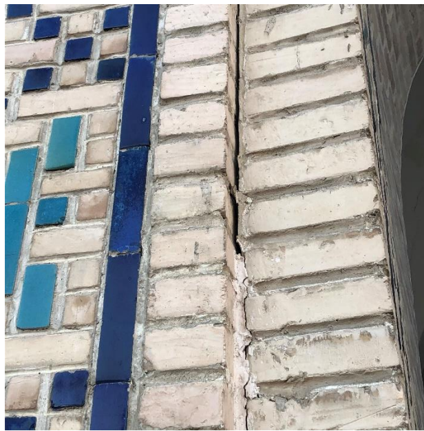
Figure 19: Kalon Mosque, evident cracking © ICOMOS/R. Mackay, 2020
