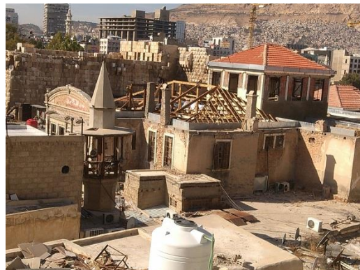
The installation of the structural system which consists of metal pillars and wooden beams for the pitched roof in the Ottoman Bank
