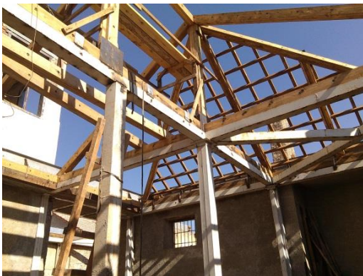
The installation of the structural system which consists of metal pillars and wooden beams for the pitched roof in the Ottoman Bank
