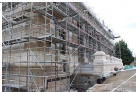
Buda Castle, Riding Hall ongoing reconstruction work © Jyoti Hosagrahar
