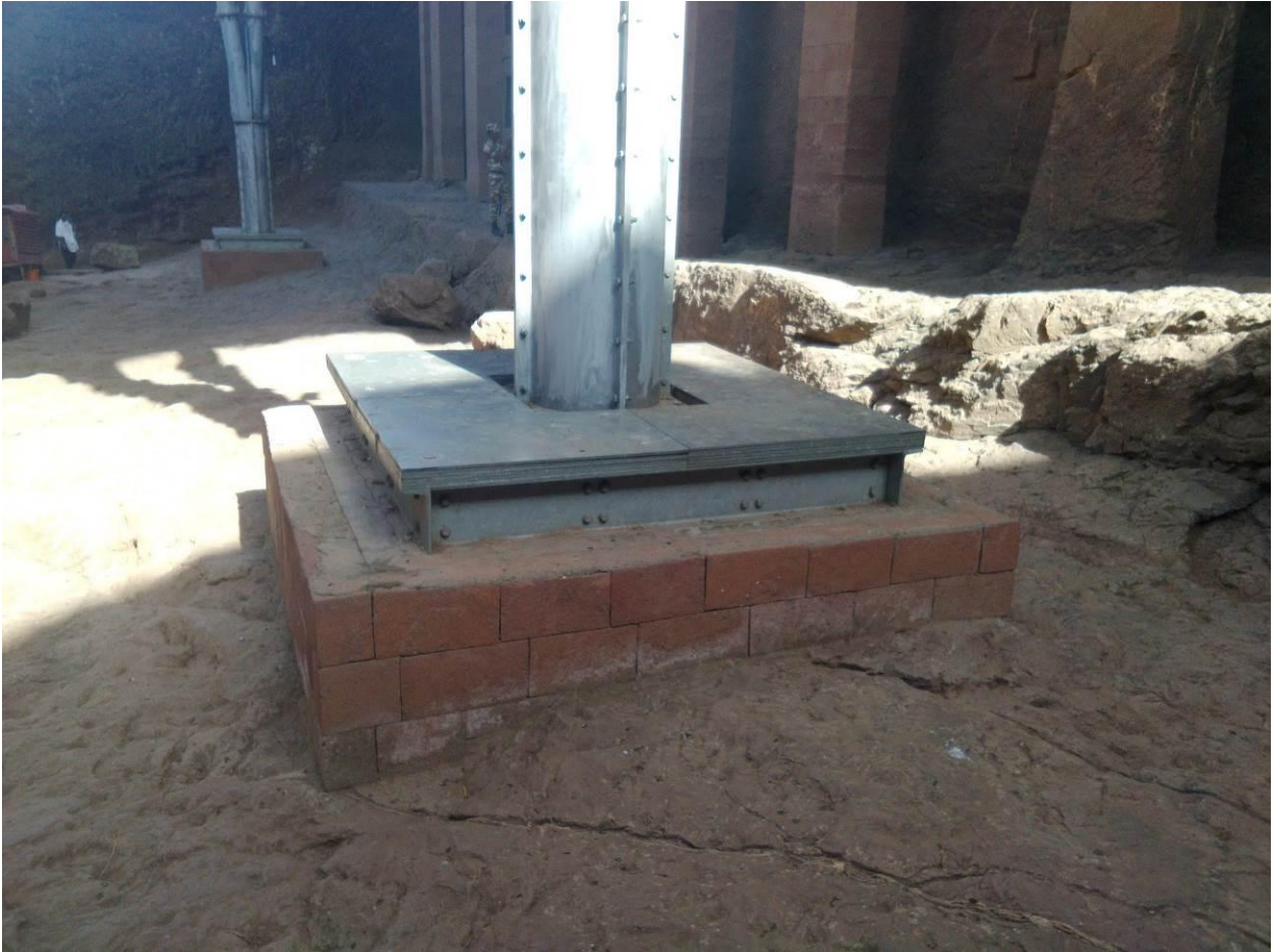
Figure 9 - Detail of pylon foundation with metal ballast plates
