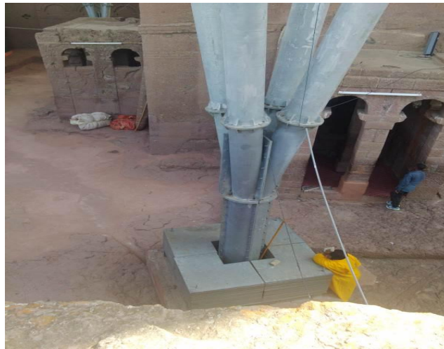
Figure 8 (a/b) – Pylons composed of individual parts bolted together and used to support the shelter construction
