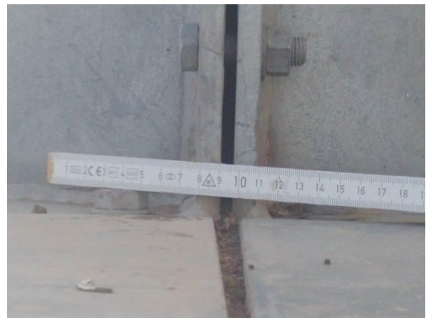
Figure 16 - (a/b/c/d) - View on the upper foundation of the shelter over Biete Abba Libanos from different angles; the roof is too short to properly drain into the (cement) lined channel and conduct of surface water is uncontrolled; some joints of the tuff stone cladding from the concrete foundation are loose, and there is an observable widening of 8mm of base steel-tube element. It is unclear if this widening has occurred during the last ten years or if it has been there from the beginning of the construction phase.
