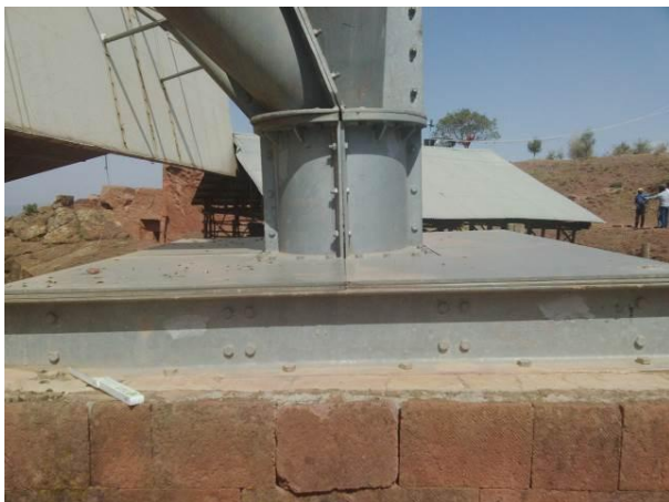
Figure 16 - (a/b/c/d) - View on the upper foundation of the shelter over Biete Abba Libanos from different angles; the roof is too short to properly drain into the (cement) lined channel and conduct of surface water is uncontrolled; some joints of the tuff stone cladding from the concrete foundation are loose, and there is an observable widening of 8mm of base steel-tube element. It is unclear if this widening has occurred during the last ten years or if it has been there from the beginning of the construction phase.
