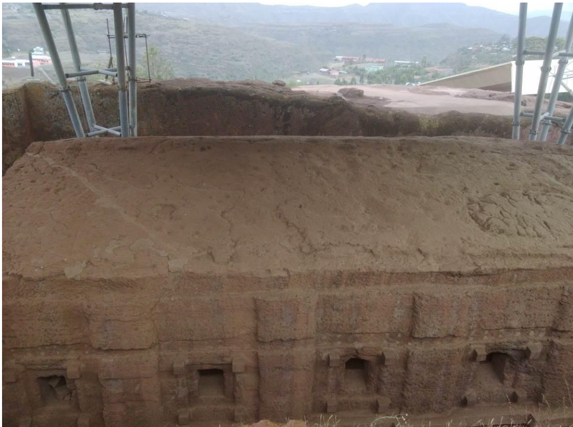
Figure 18 -Detail of roof of Biete Amanuel showing dry, dusted, fragmented surface
