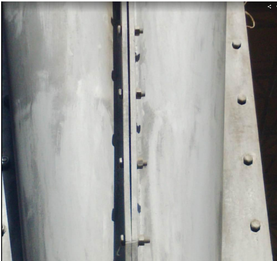
Figure 11 -Detail of upper joint of pylon showing example of the joint opening between individual tube parts
