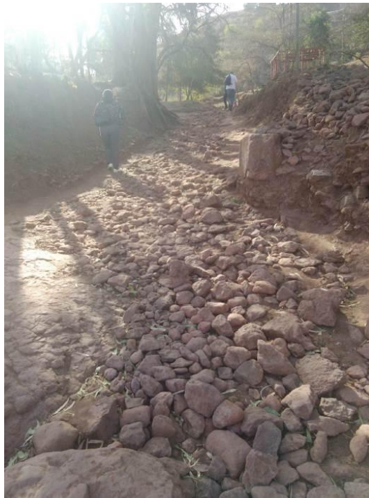
Figure 39 -Steps and pathway built as part of the World Bank project but no longer maintained in large areas
