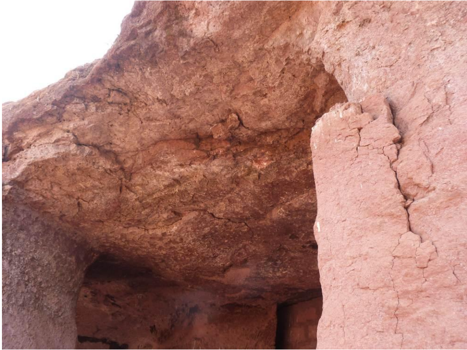
Figure 30 -Example of decayed stone prone to detachment in Biete Mekerios
