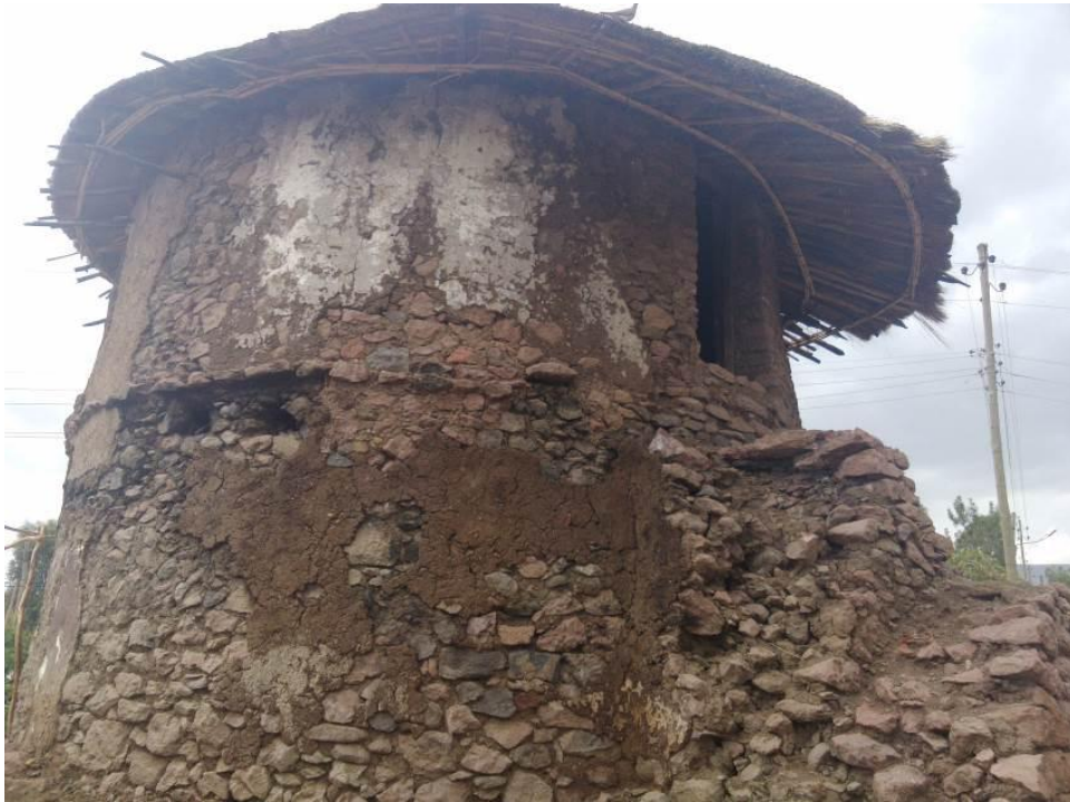
Figure 38 - Dilapidating traditional "tukul" house construction; a comprehensive survey on the location and condition of the remaining houses is needed.
