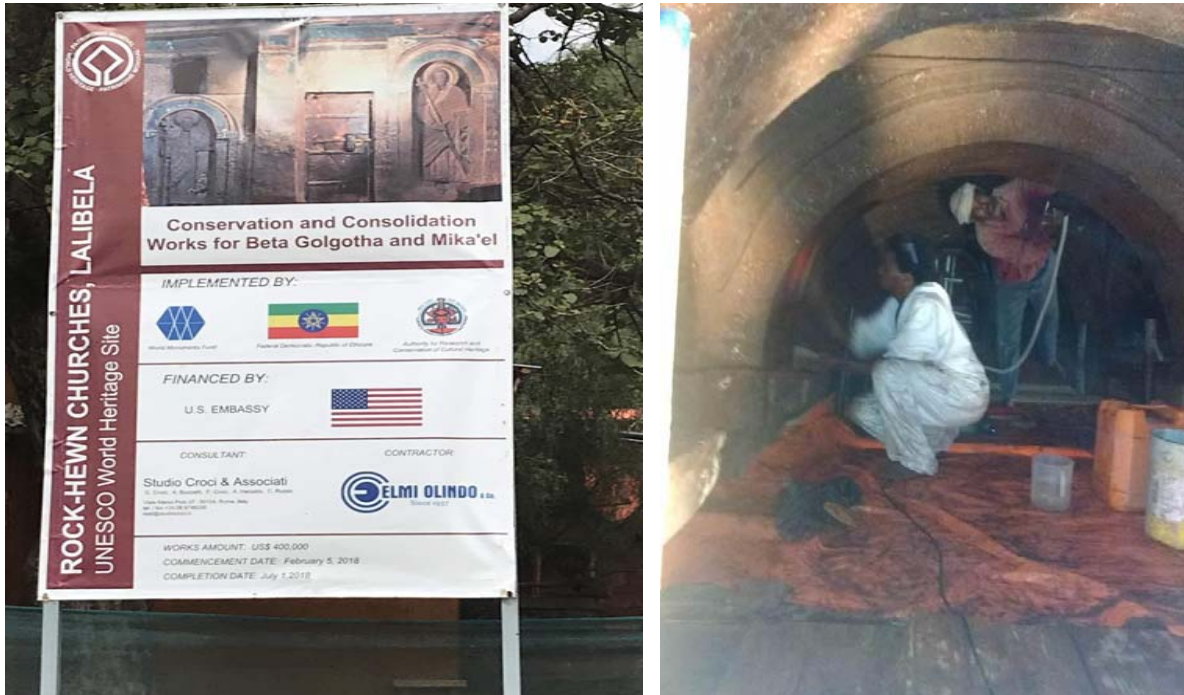
Figure 22 - (a) - Recent conservation work (ongoing) implemented in partnership between Ethiopian authorities and World Monuments Fund and financed by the US Ambassadors Fund – (b) Details of surface cleaning works being carried out as part of the current conservation programme at Biete Golgotha Mikael
