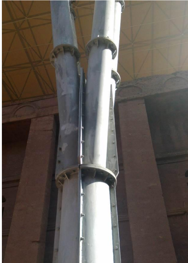
Figure 10 -Upper joint of a pylon at Biete Medhane Alem
