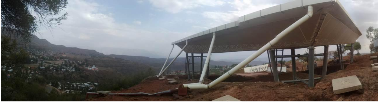
Figure 19 -Unmaintained drainage system from the shelter over Biete Amanuel
