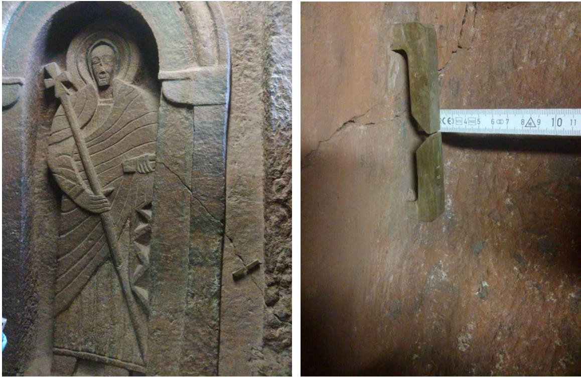
Figure 24 -Carved effigy in Biete Golgotha with one of the Angelini gauges inserted in 1968 to monitor the discontinuity in the rock; all inspected gauges in this area showed deformations of less than 3mm.
