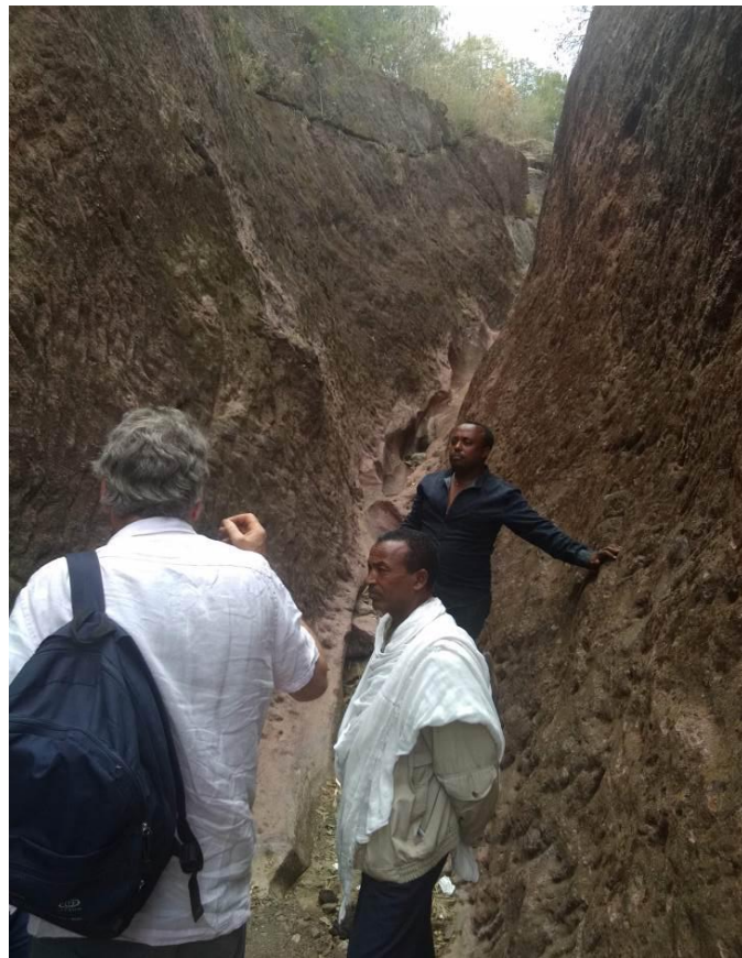
Figure 29 – Experts inspecting the original drainage ditches below Biete Ghiorgis. The function of this system is not fully investigated and understood. Its complete excavation has been suggested in previous reports, resulting in the creation of cavities that capture water in some areas instead of draining it. Excavations of these systems require topographical and archaeological study to evaluate the extent to which the “original” shape (considered to be the native rock bed) is suitable for drainage purposes.
