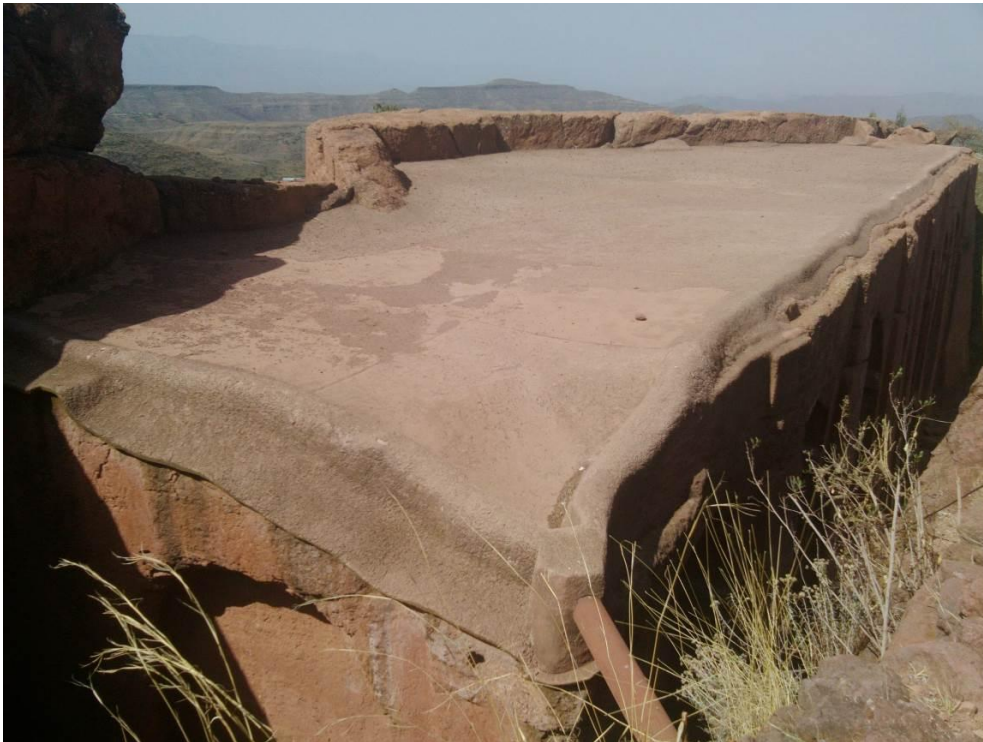
Figure 13 -Roof of Biete Gabriel re-covered as part of the conservation programme of works completed in 2016 by World Monuments Fund and Studio Croci
