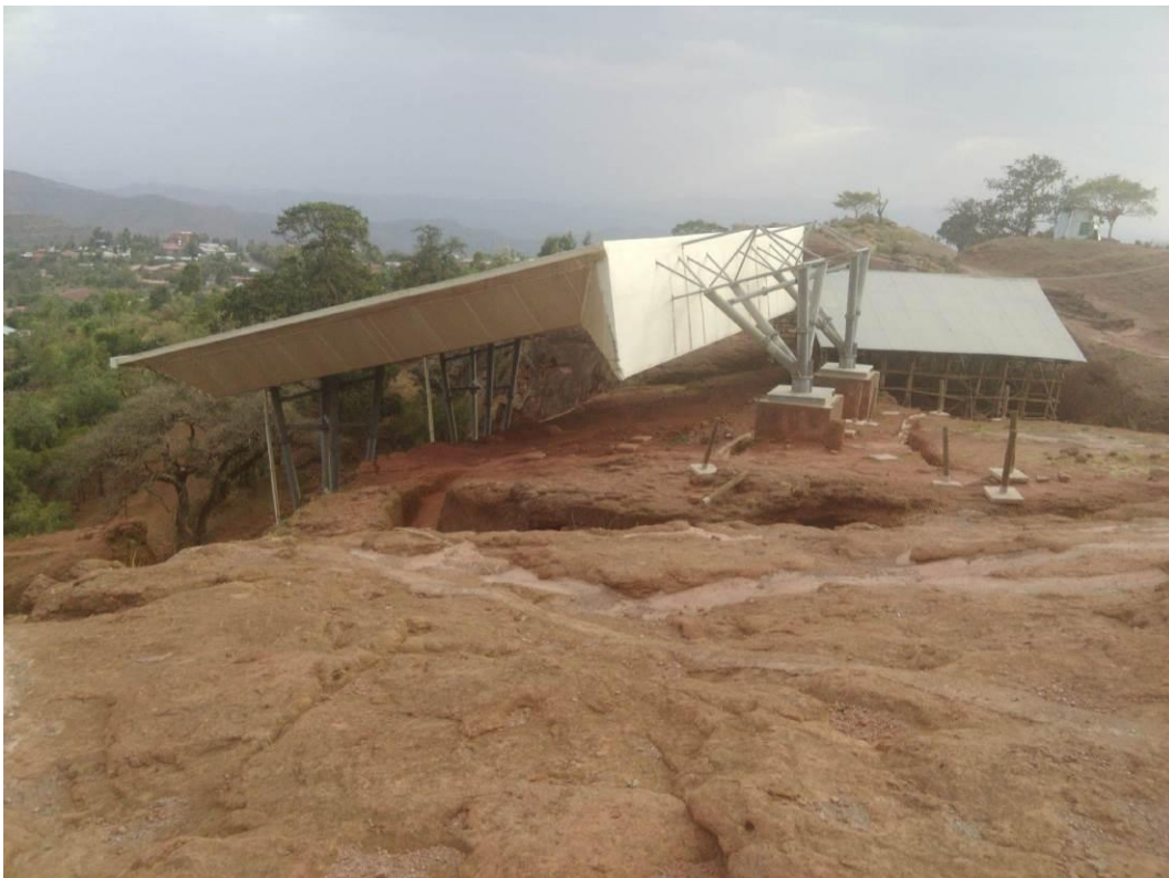
Figure 15 -View of shelter over Biete Libanos from the upper side; note the slope of the topography directing surface waters towards the cliff's edge
