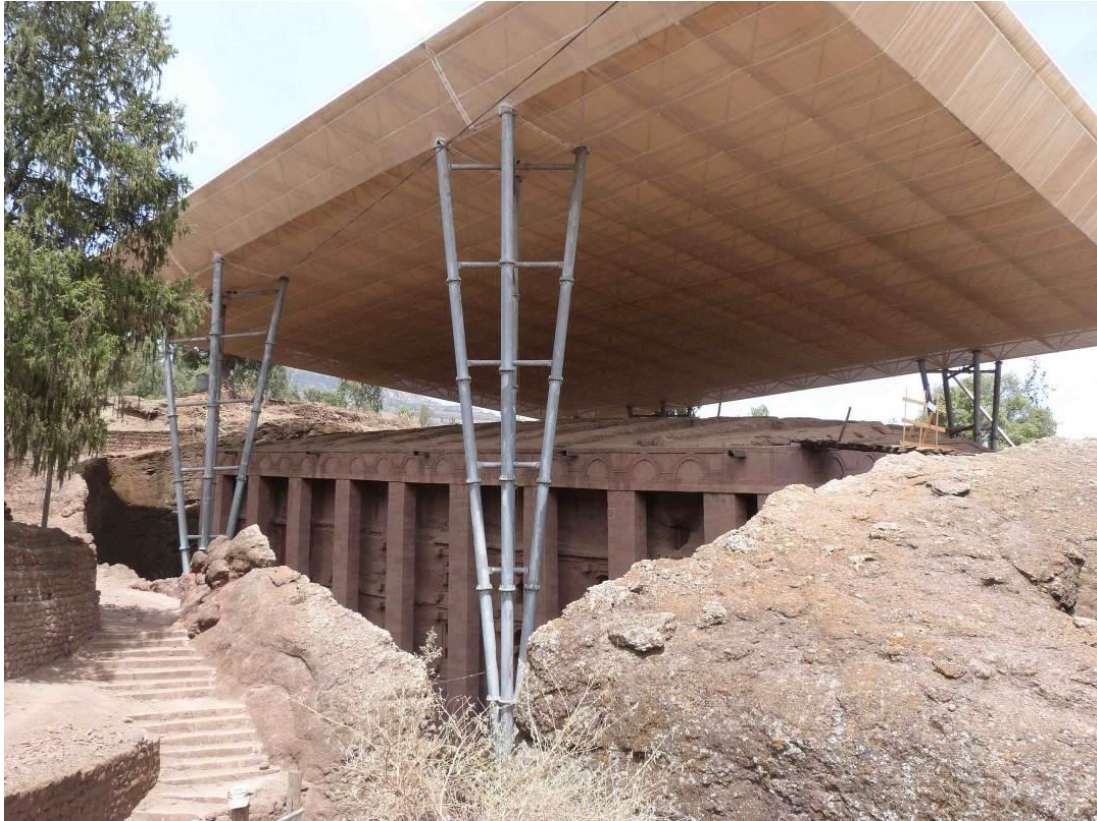
Figure 3 - Modern shelter for Biete Medhane Alem erected in 2007
