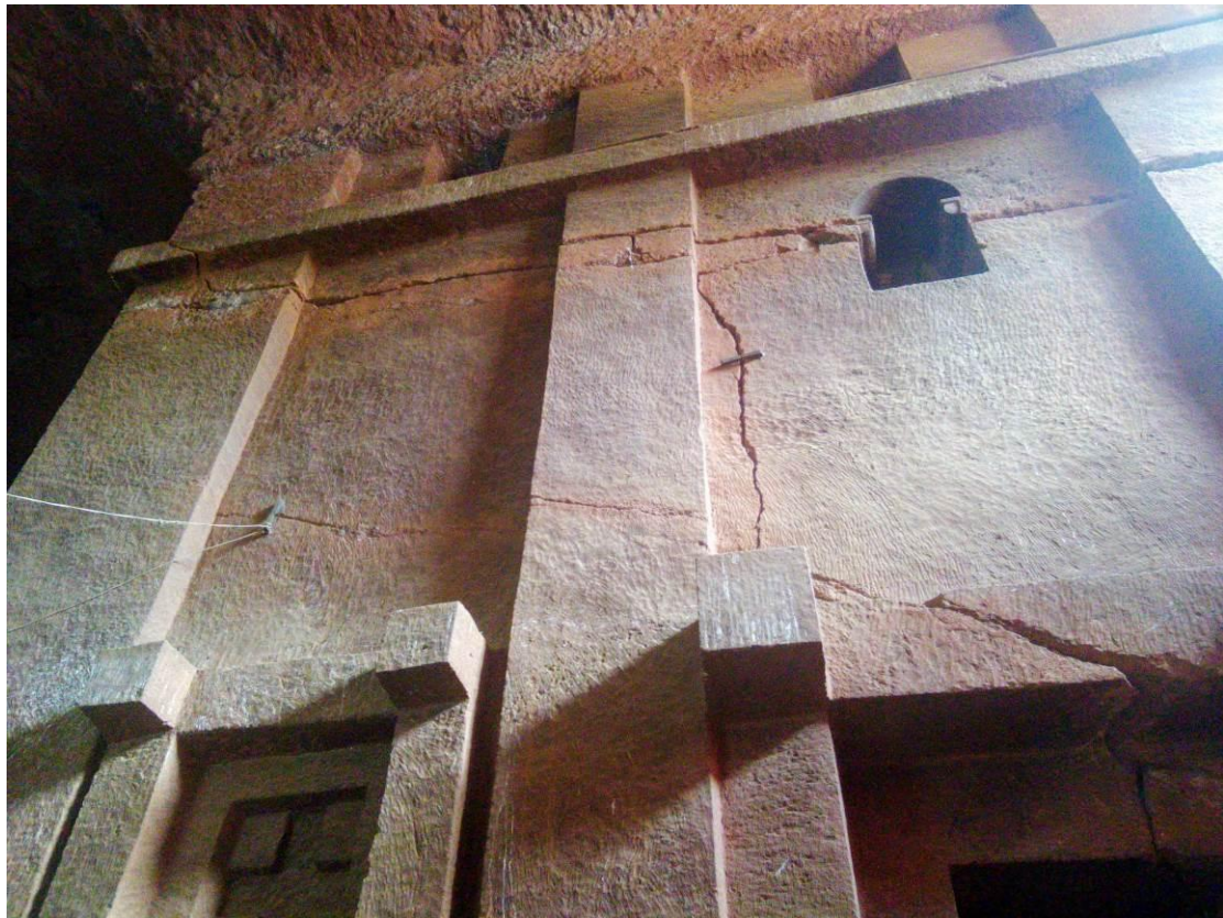
Figure 25 -Rock discontinuities on the side elevation of Biete Abba Libanos; note the gauges installed by Angellini in 1968, most of these gauges require a ladder or some type of simple scaffolding for proper reading.
