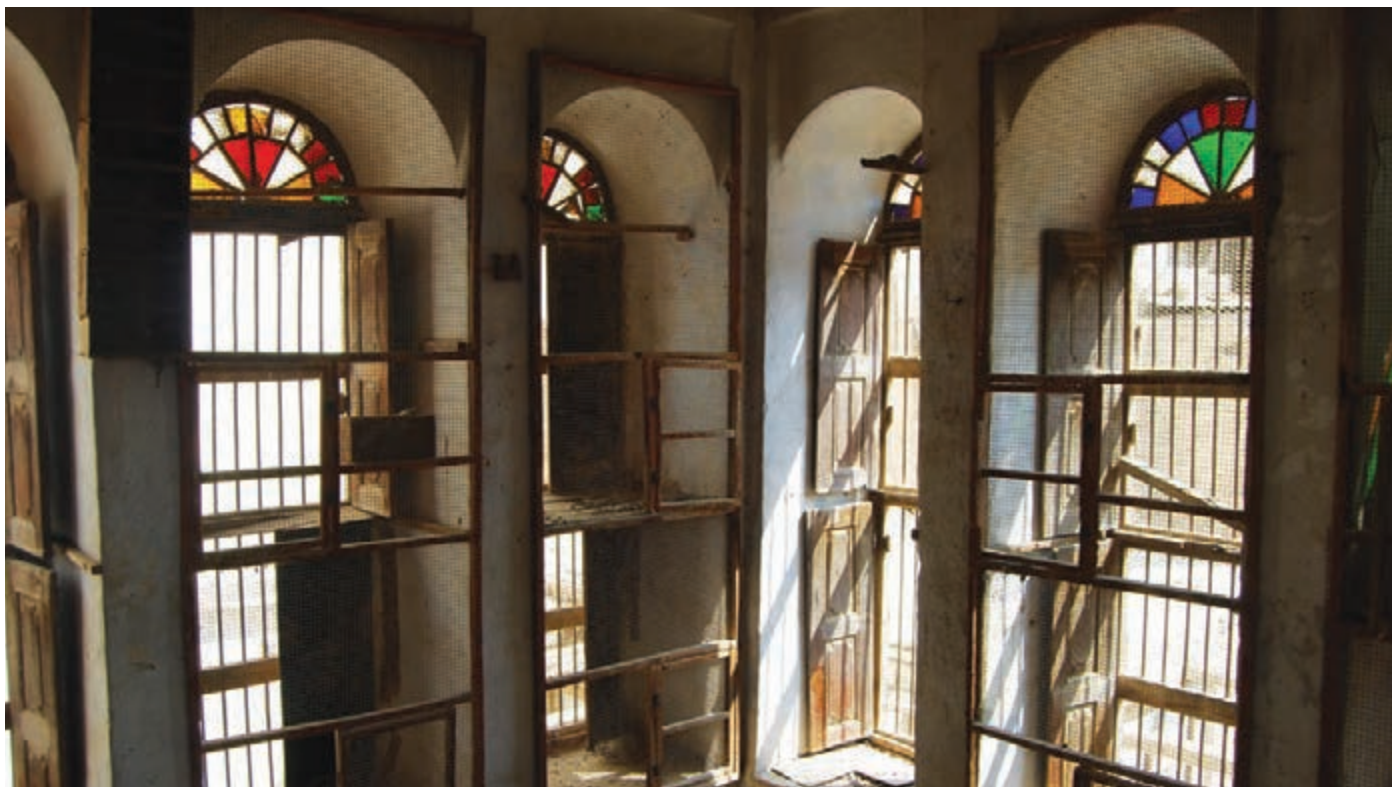
Details of window frames in Al-Jalahma House
