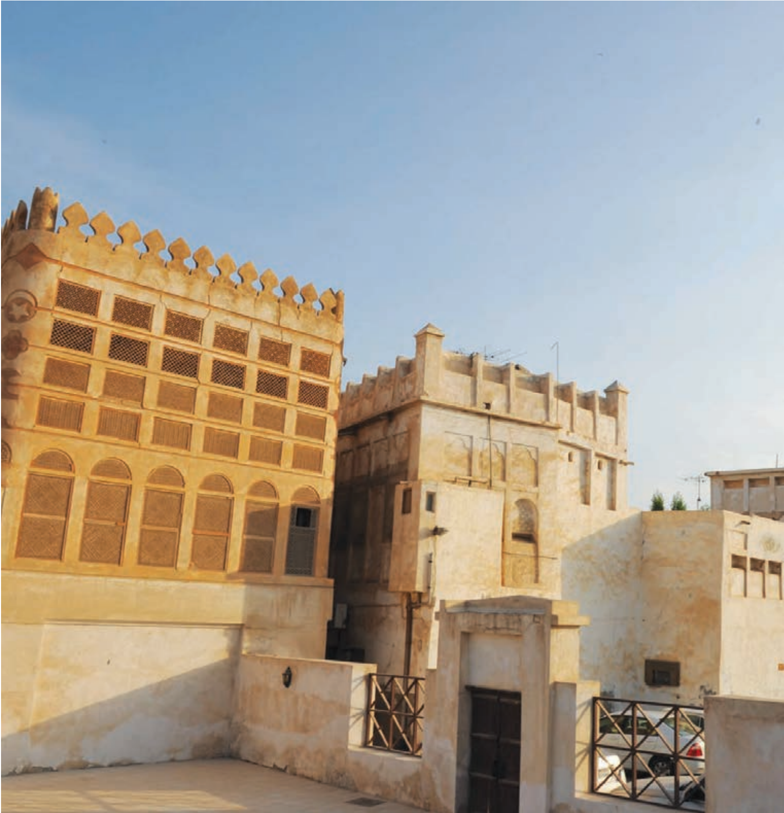
Southern façade of Siyadi complex from courtyard of Siyadi Mosque
