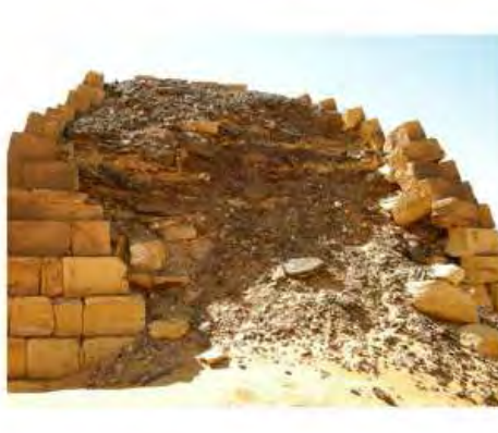
DSCN3742.JPG, Structural Deterioration of Pyramids, Northern Cemetery
