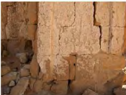
DSCN4151.JPG, Naqaa, Temple F, Exposure and Deterioration of Ancient Plasters, Structural Instability of Walls/Collapse of Archaeological Features, Structural Instability of Walls/Collapse of Archaeological Features
