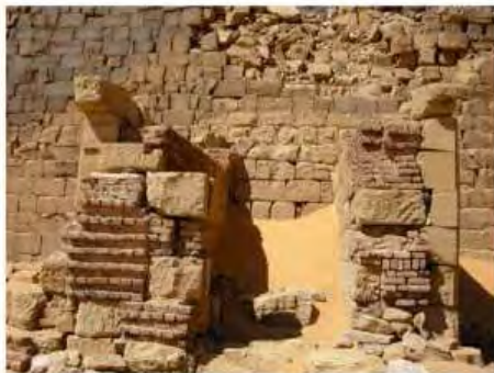
DSCN3763.JPG, Incoherent Repair Methods and Poor Craftmanship, Northern Cemetery
