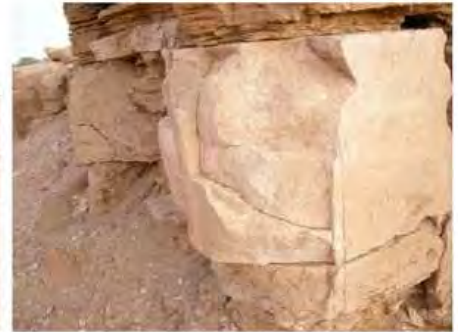
DSCN3958.JPG, Degradation of Stone/Masonry Elements, Structural Instability of Walls/Collapse of Archaeological Features, Royal City
