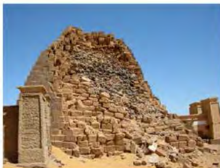
DSCN3802.JPG, Structural Deterioration of Pyramids, Southern Cemetery
