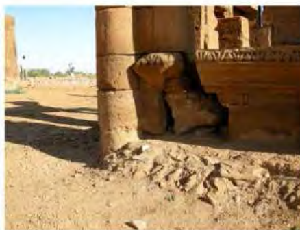
DSCN4003.JPG, The Kiosk - Naqaa, Naqaa, Degradation of Stone/ Masonry Elements, Inappropriate/Inexistent Site Drainage
