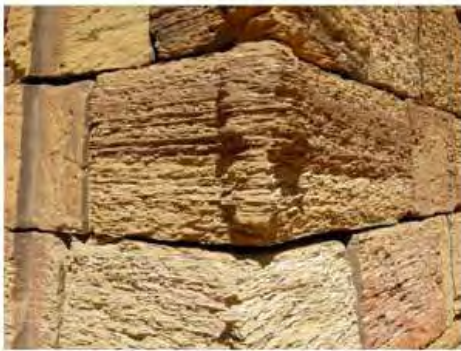
DSCN3750.JPG, Degradation of Stone/Masonry Elements, Northern Cemetery
