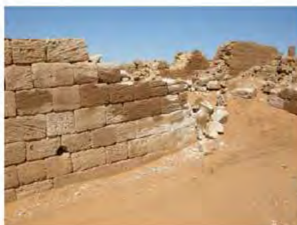
DSCN4171.JPG, Musawwarat - Great Enclosure, Degradation of Stone/Masonry Elements, Structural Instability of Walls/Collapse of Archaeological Features, Structural Instability of Walls/Collapse of Archaeological Features, Salt Crystallization
