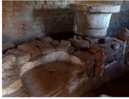
DSC06269.JPG, Inappropriate/Inexistent Site Drainage, Degradation of Stone/Masonry Elements, Exposure and Deterioration of Ancient Plasters, Royal City
