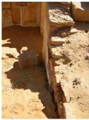
DSCN4120.JPG, Naqaa, Amun Temple, Exposure and Deterioration of Ancient Plasters, Inappropriate/Inexistent Site Drainage
