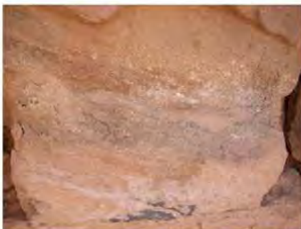
DSCN4005.JPG, The Kiosk - Naqaa, Naqaa, Degradation of Stone/ Masonry Elements, Inappropriate/Inexistent Site Drainage
