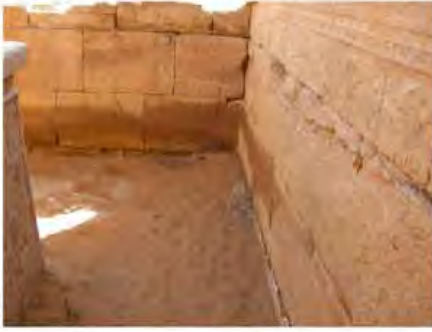
DSCN4127.JPG, Naqaa, Amun Temple, Inappropriate/Inexistent Site Drainage, Water Damage, Degradation of Stone/Masonry Elements
