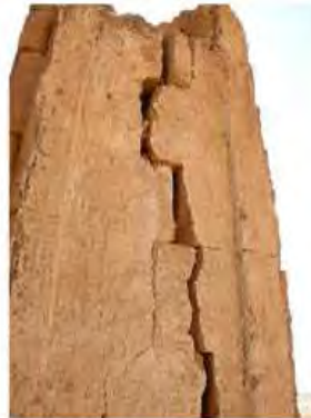
DSCN4152.JPG, Naqaa, Temple F, Structural Instability of Walls/Collapse of Archaeological Features, Exposure and Deterioration of Ancient Plasters, Structural Instability of Walls/Collapse of Archaeological Features
