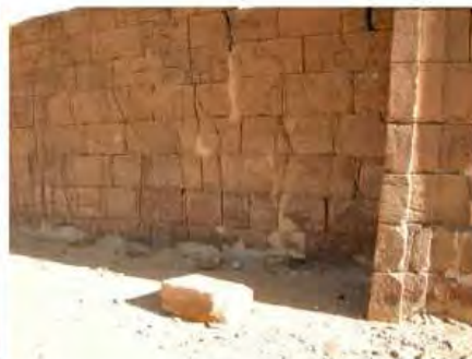
DSCN4029.JPG, Lion Temple B300 - Naqaa, Naqaa, Degradation of Stone/Masonry Elements, Inappropriate/Inexistent Site Drainage
