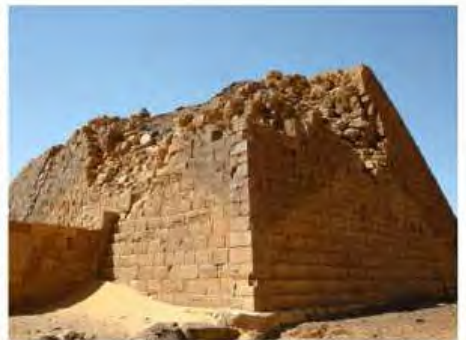
DSCN3764.JPG, Structural Deterioration of Pyramids, Northern Cemetery
