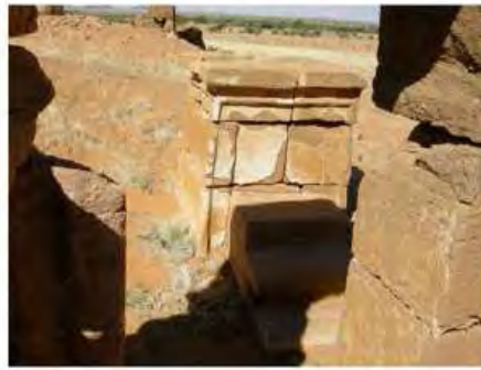
DSCN4123.JPG, Naqaa, Amun Temple, Exposure and Deterioration of Ancient Plasters, Inappropriate/Inexistent Site Drainage
