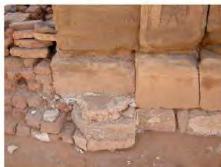
DSCN4094.JPG, Naqaa, Amun Temple, Degradation of Stone/ Masonry Elements, Exposure and Deterioration of Ancient Plasters
