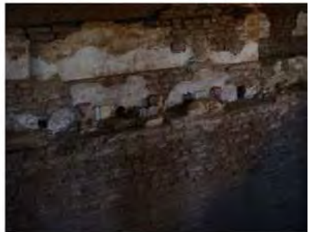
DSC06254.JPG, Exposure and Deterioration of Ancient Plasters, Degradation of Stone/Masonry Elements, Inappropriate/Inexistent Site Drainage, Royal City
