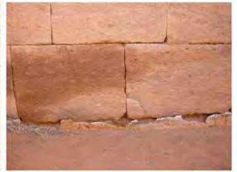
DSCN4129.JPG, Naqaa, Amun Temple, Exposure and Deterioration of Ancient Plasters, Inappropriate/Inexistent Site Drainage
