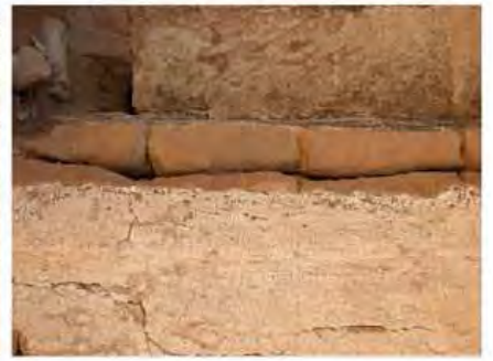
DSCN4153.JPG, Naqaa, Temple F, Exposure and Deterioration of Ancient Plasters, Water Damage
