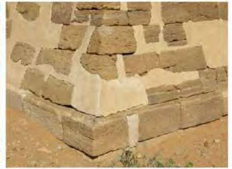
DSCN3832.JPG, Unsympathetic Repair Work/Interventions, Southern Cemetery
