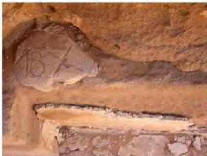
DSCN4093.JPG, Naqaa, Amun Temple, Exposure and Deterioration of Ancient Plasters, Degradation of Stone/Masonry Elements
