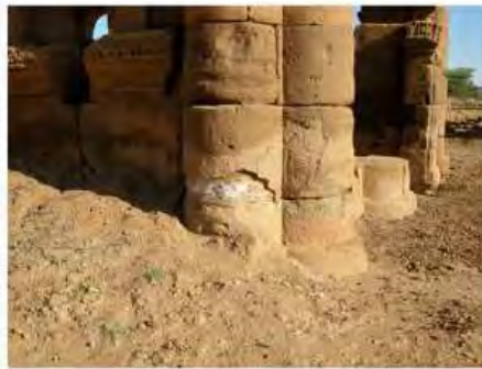
DSCN4000.JPG, The Kiosk - Naqaa, Naqaa, Degradation of Stone/ Masonry Elements, Inappropriate/Inexistent Site Drainage
