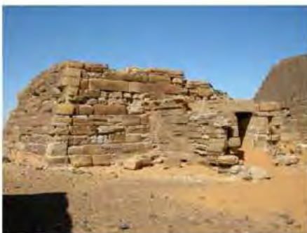
DSCN3726.JPG, Degradation of Stone/Masonry Elements, Northern Cemetery
