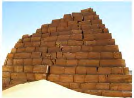
DSCN3740.JPG, Structural Deterioration of Pyramids, Northern Cemetery
