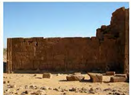
DSCN4030.JPG, Lion Temple B300 - Naqaa, Naqaa, Degradation of Stone/Masonry Elements, Inappropriate/Inexistent Site Drainage
