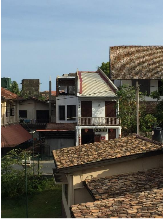
Fig. 16 An example of illegal development
