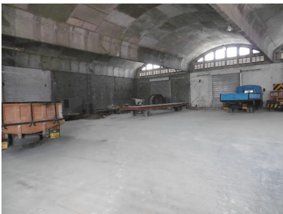
Fig. 3 Interior of warehouse
