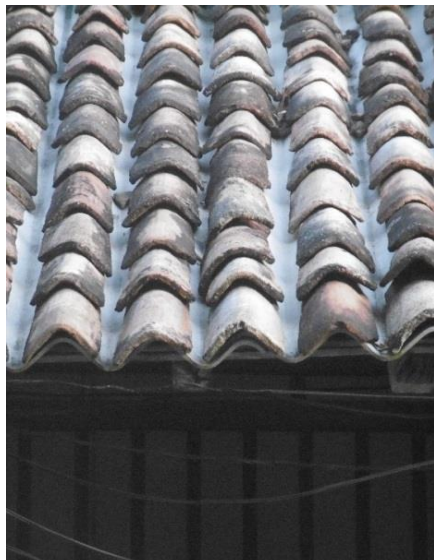
Fig. 11 Asbestos sheet under clay tiles
