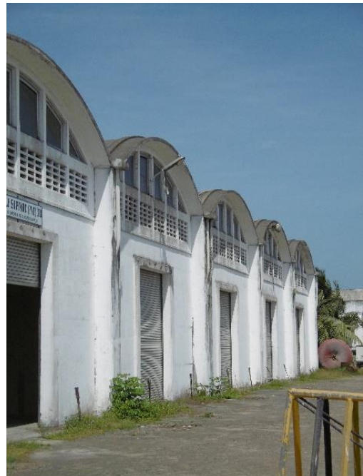
Fig. 2 Part of the range of the warehouses
