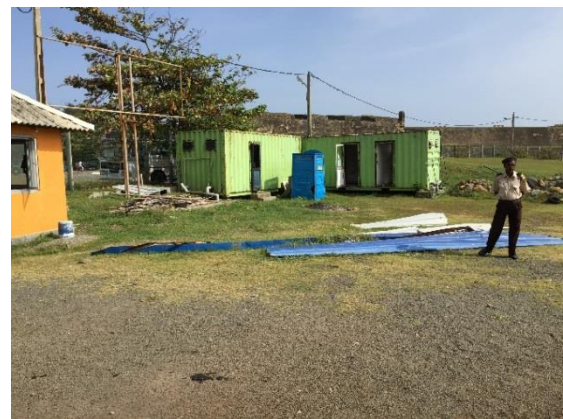
Fig. 8 Temporary building housing changing facilities
