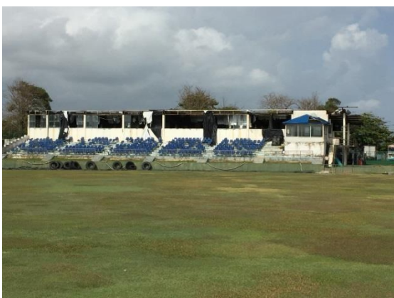
Fig. 7 The semi-ruined building housing indoor cricket nets
