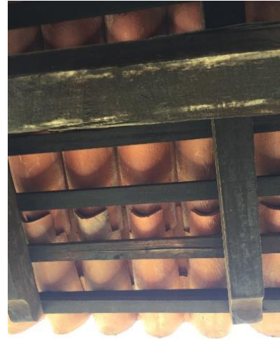
Fig. 10 Modern version of traditional tiles seen from below
