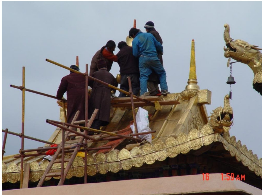
Fig.1 Traditional gilt bronze techniques applied for conservation and renovation of the Golden Top of Potala Palace
