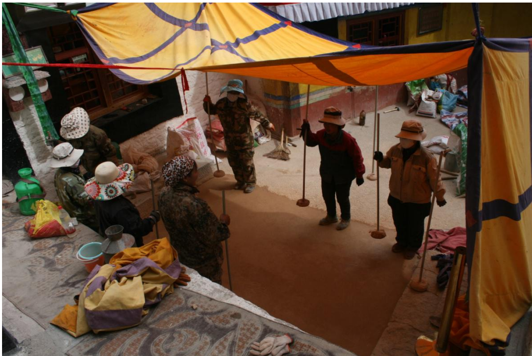
Fig. 2 Traditional ramming skills applied for maintenance of the a-ga clay on the roof surface of Xuecheng City Complex
