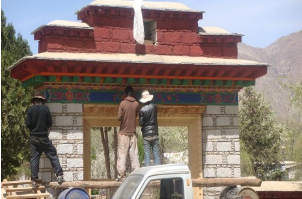
Fig. 3 Making of door-curtain of ancient building at Norbulingka
