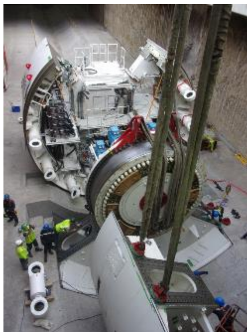
Imagen IX.2. Quito Metro tunnel boring machine being assembled
