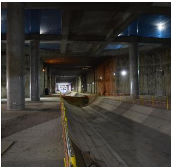
Imagen IX.1. Slurry walls constructed at the El Labrador Station, mezzanine level.
