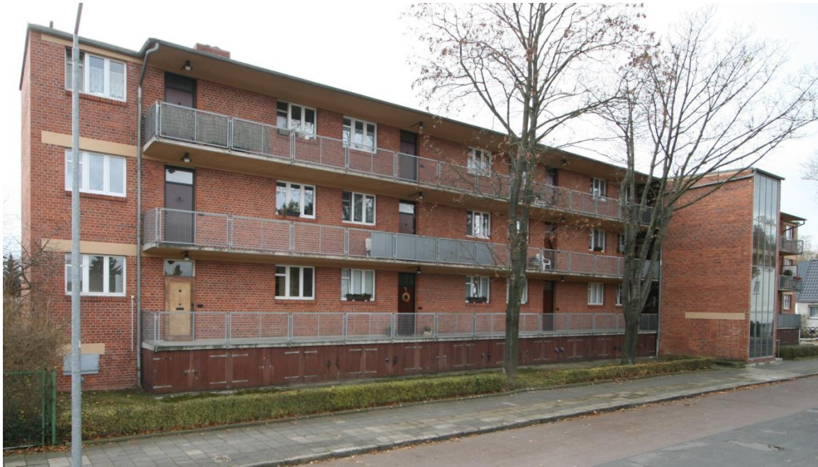
Houses with Balcony Access
