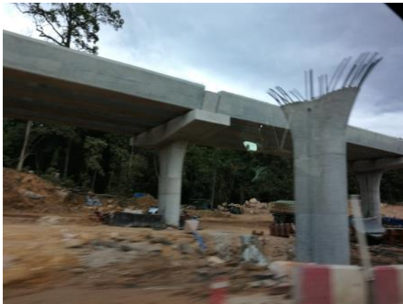
Image 8: Construction of an overpass as part of the expansion of Highway 304.
